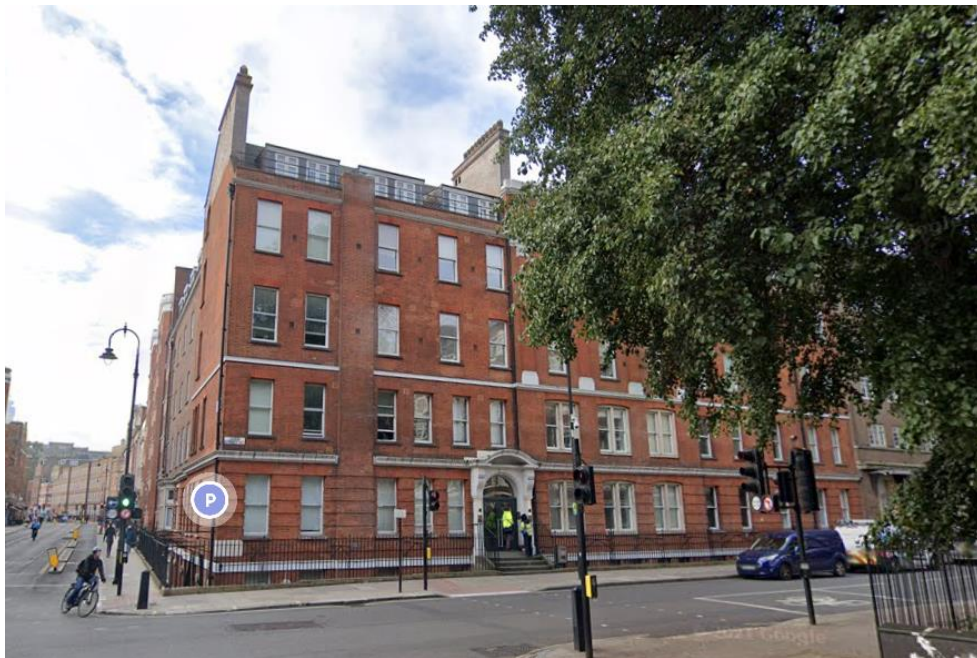
Site viewed from Tavistock Place (east)
