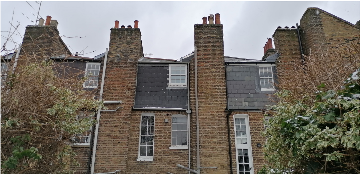
Photo 11. Rear elevation showing non-original 2nd floor sash window within slates. We aim to reinstate the original proportions of this window as still extant on the two adjacent houses.
