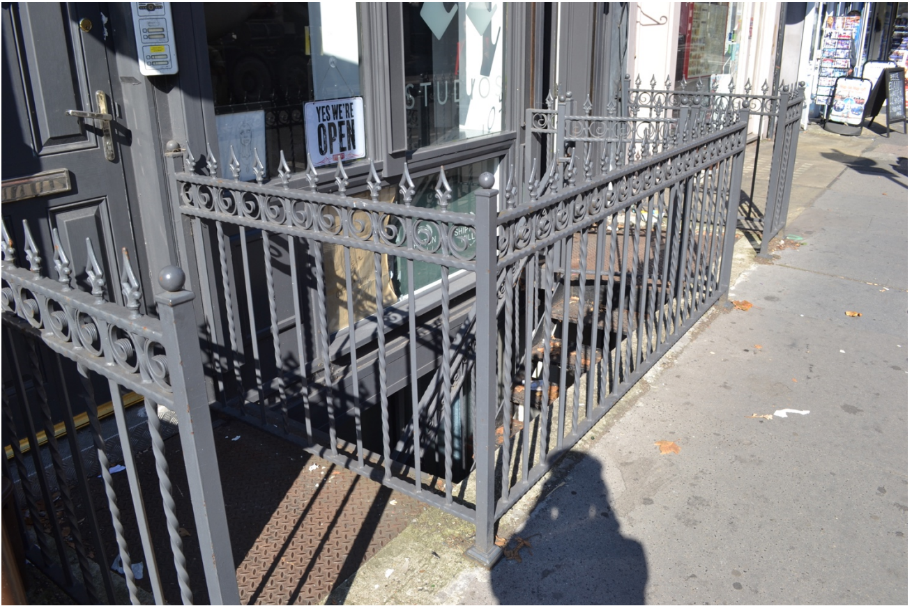
Above: Inappropriate design quality of railings. Mild steel checker plates at ground level. Railings affixed to pavement. Glazing is visible at stall riser level
