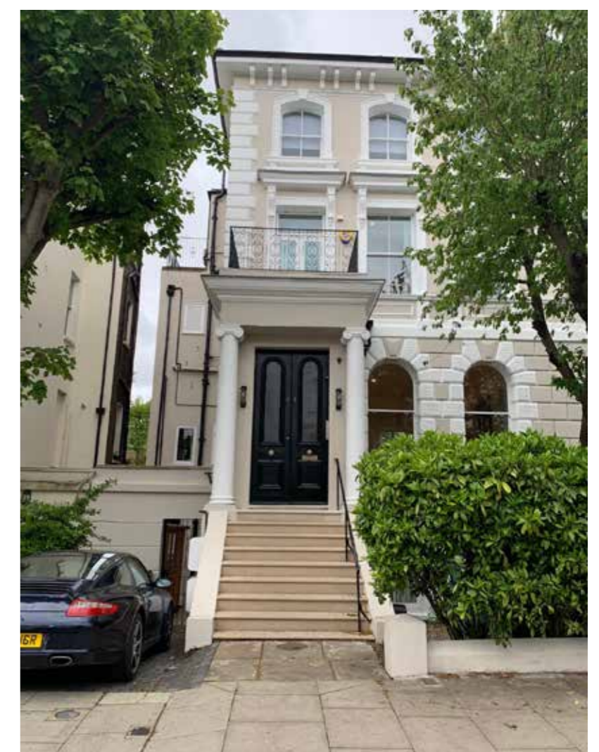
Existing Front 29 Buckland Crescent
