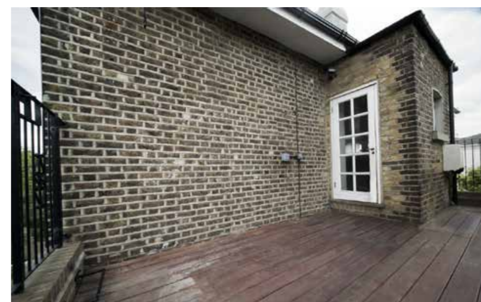
View from existing terrace towards kitchen door
