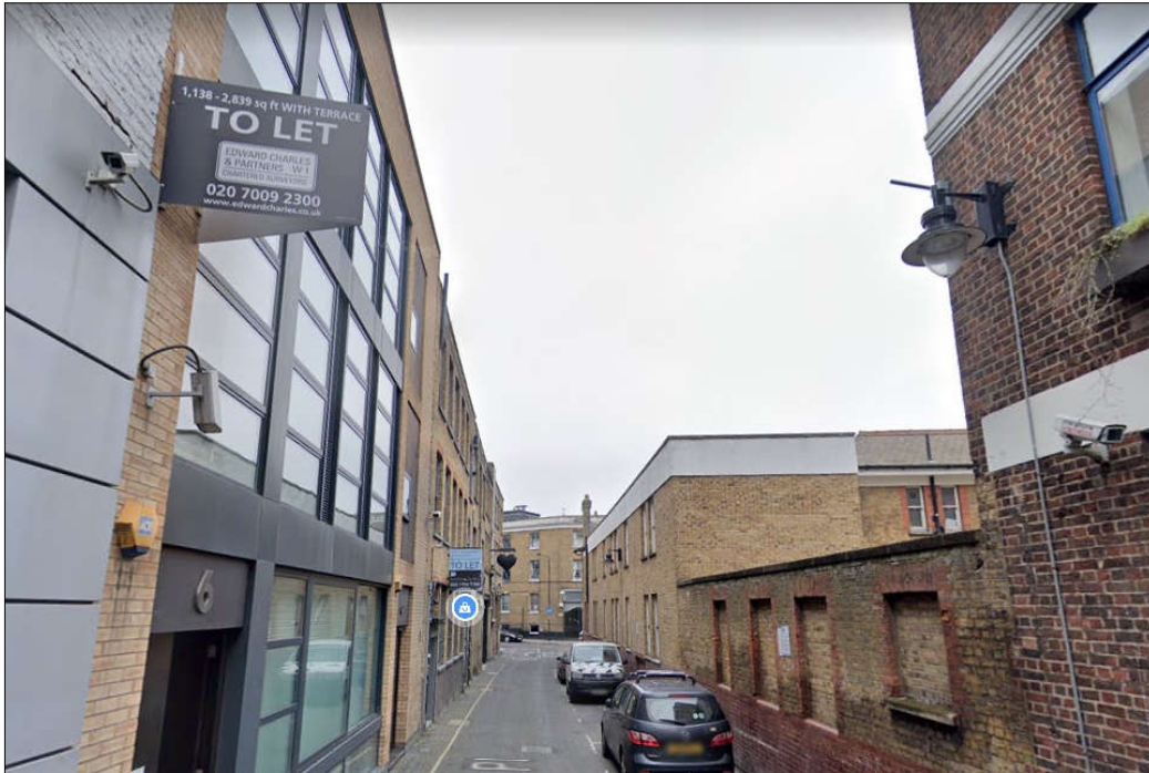
Figure 4 – Existing Highway overhangs to Greenland Place
