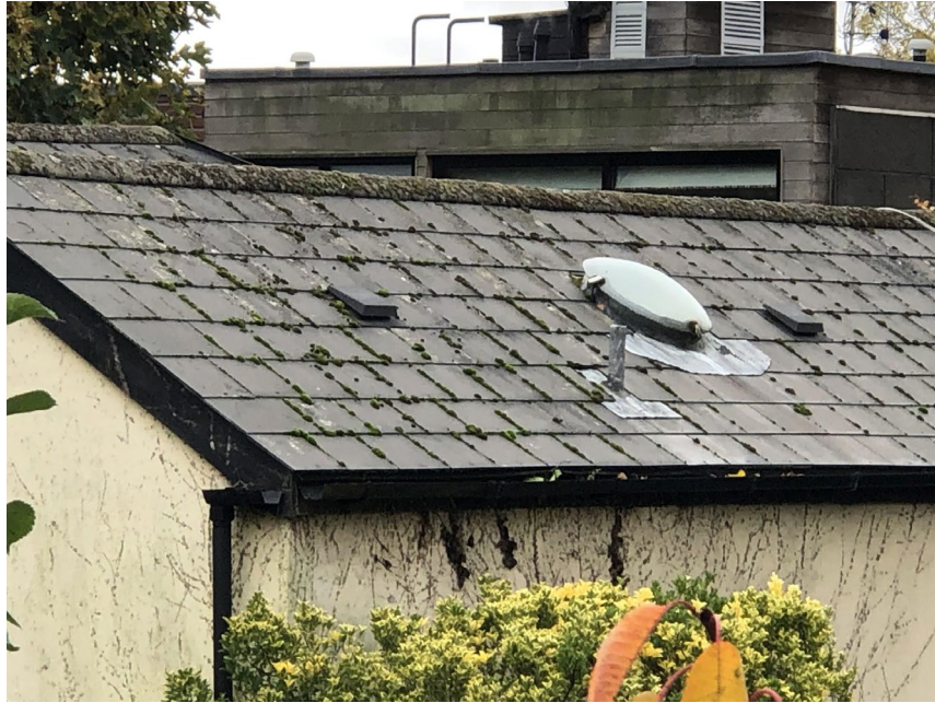
Existing roof tiles for house no.1 - Example 2.
