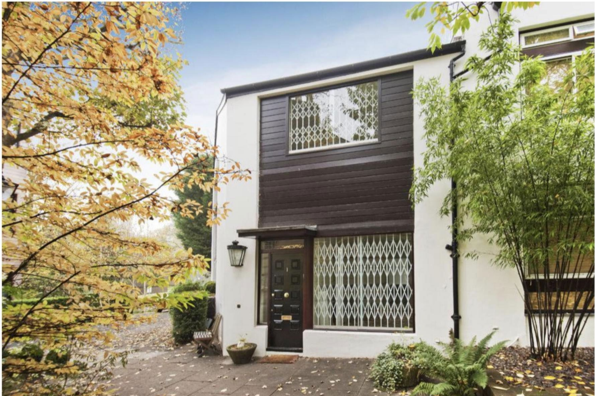
Elevated side view of 1 and 2 Oak Hill Park Mews
