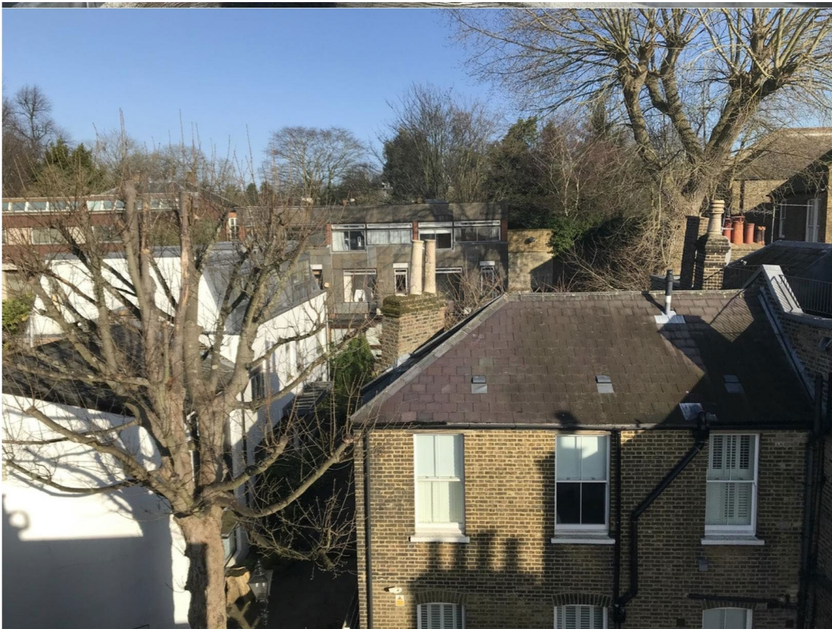
Elevated side view of 1, 2 and 3 Oak Hill Park Mews
