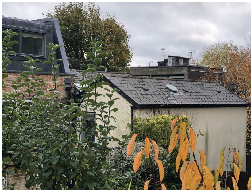
Existing roof tiles of house no.1 - Example 1
