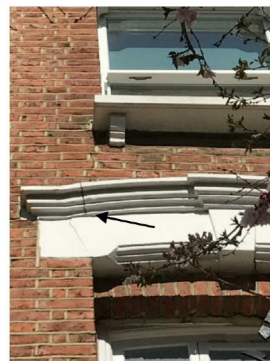
Cracking to front elevation
