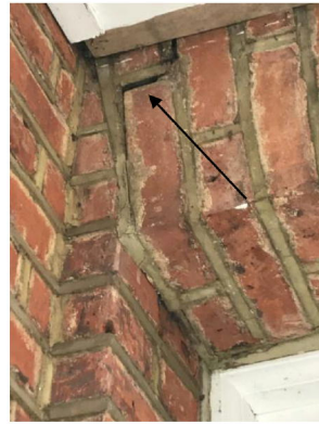
Cracking above front door arch
