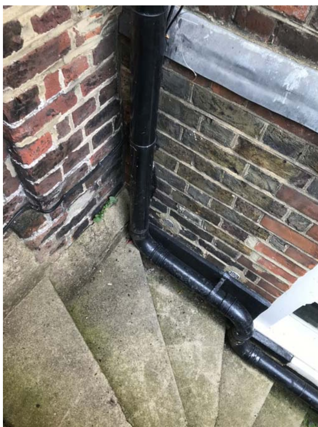
Figure 8 plastic rainwater pipe with Doulton tubes above
