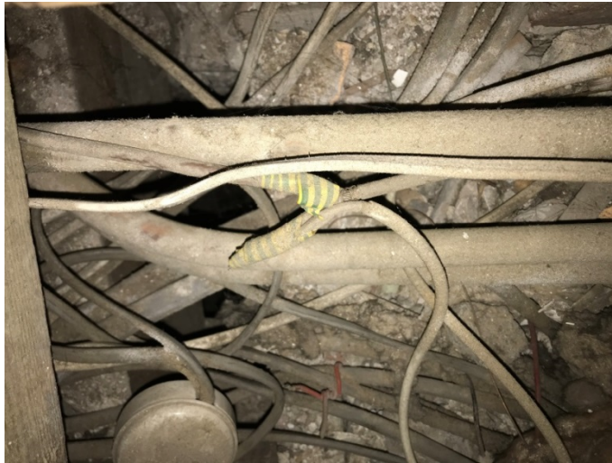
Figure 2 Typical services beneath the floorboards
