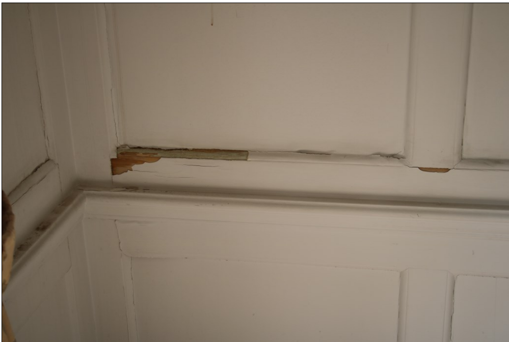
Photograph 5: Detail of panelling in left hand room -note the paint chip and lack of paint layers and the brightness of the pine exposed Photograph by the author
