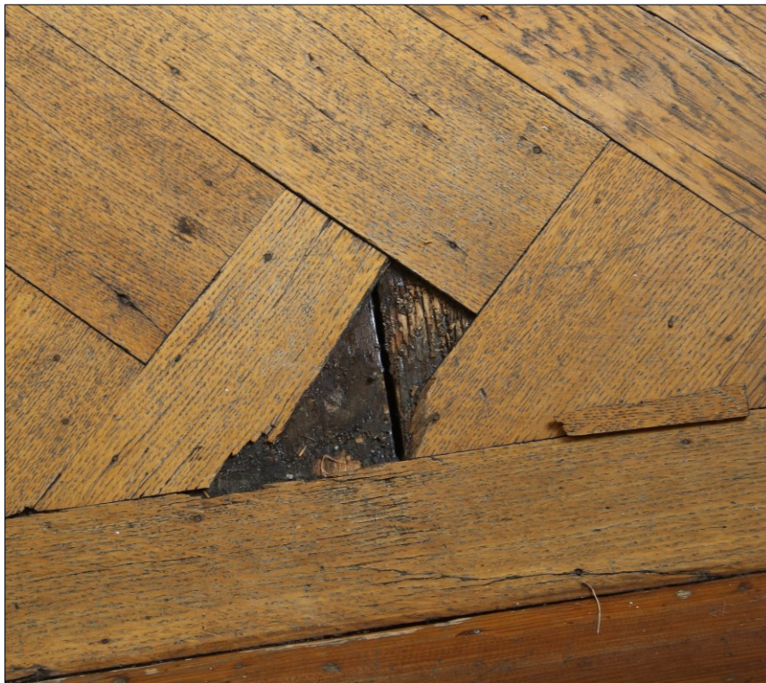
Photograph 8: Detail of parquet veneer at threshold to right hand room ground floor- note small section of painted or stained timber exposed below having the character and appearance of early 20 th date Photograph by the author
