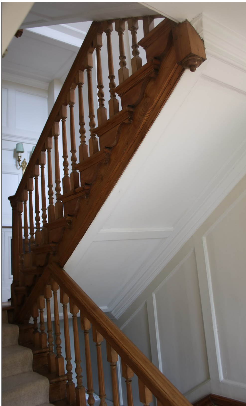
Photograph 3: Main stair dog leg return showing the ground floor and first floor flights – note the open or cut string and the simple but elegant modillion moulding to the tread ends which are visible on the first-floor flight. These are also visible on the ground-floor flight from the hall Photograph by the author
