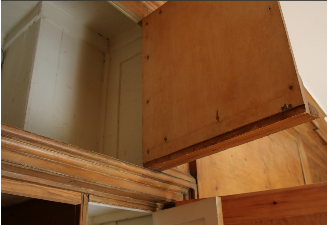
Photograph 4: Right hand ground floor room detail of panelling to the cupboard by the fireplace – note the simple painted panelling inside the cupboard and the more elaborate waxed panelling in the room with the matching panel planted onto the cupboard door. The lower section of the planted panel has been created with great care to replicate the architrave below and therefore when closed to be almost invisible; a “jib” door Photograph by the author
