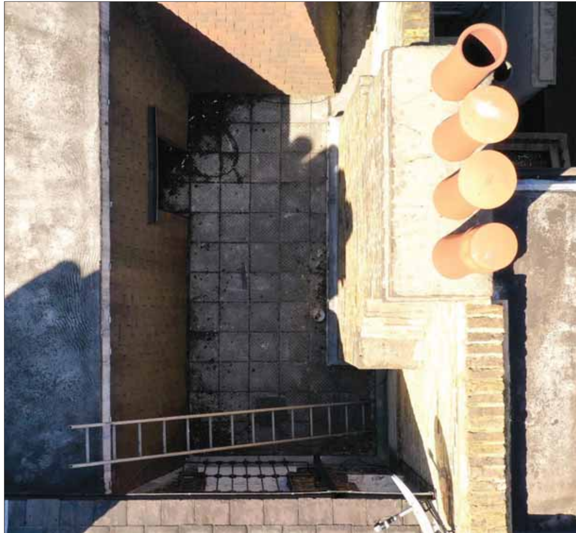
Image 9: Roof 4 Covered with Non-slip Tiles.
