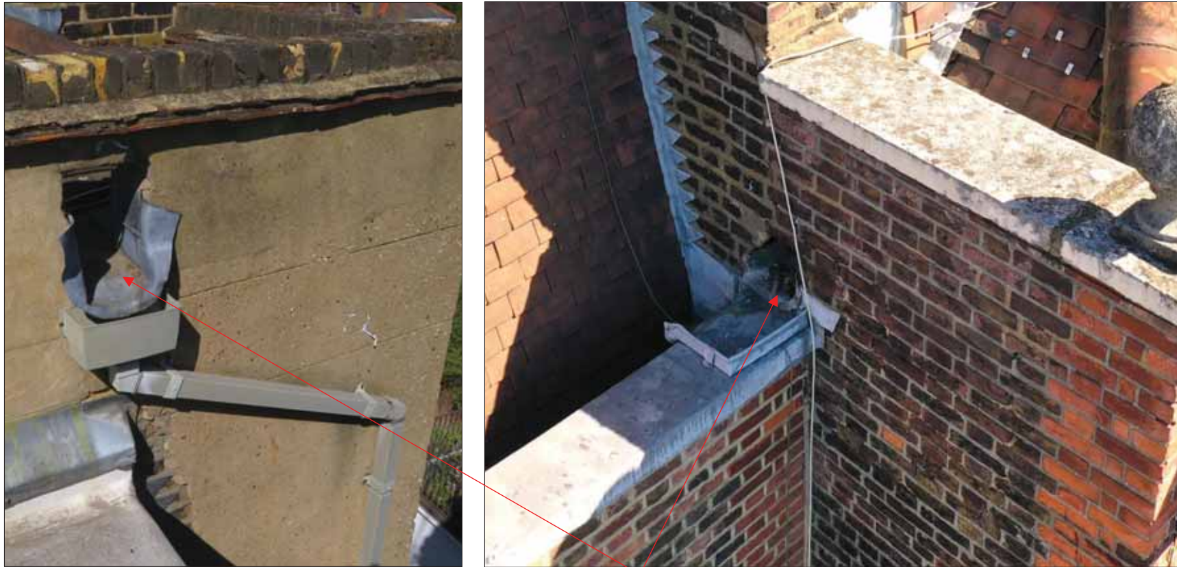
Images 27 & 28: Example Areas Where Rainwater from Neighbouring Properties Flows into the System of 5 Elm Row.
