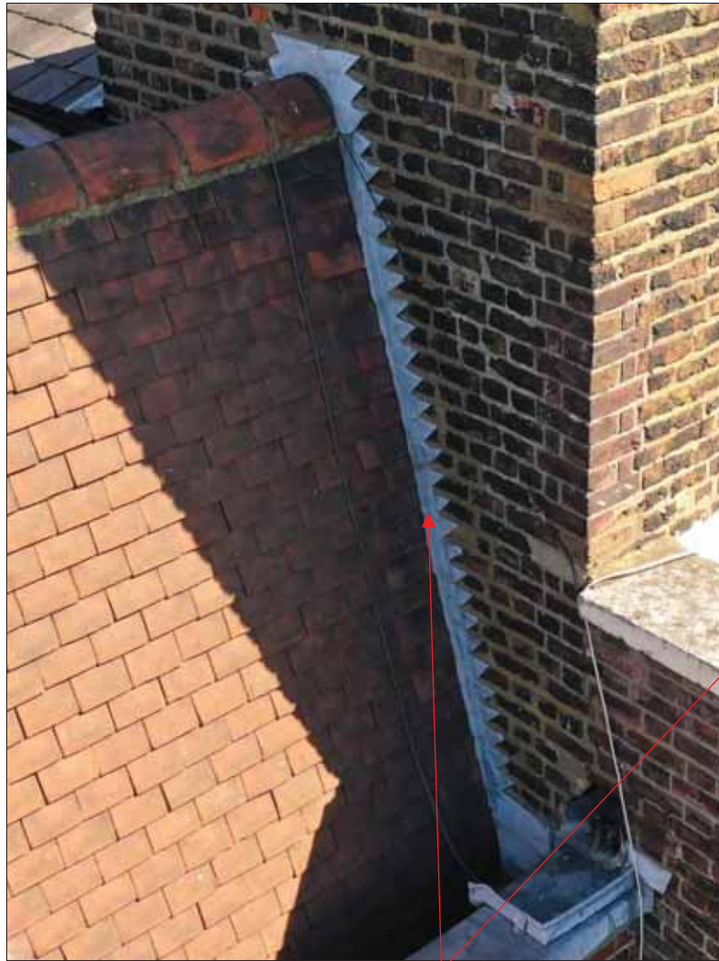
Images 17 & 18: Example Areas of Older Leadwork to the East Party Wall & Top of the Mansard, Note the Newer Leadwork to Stack 1 Adjacent.
