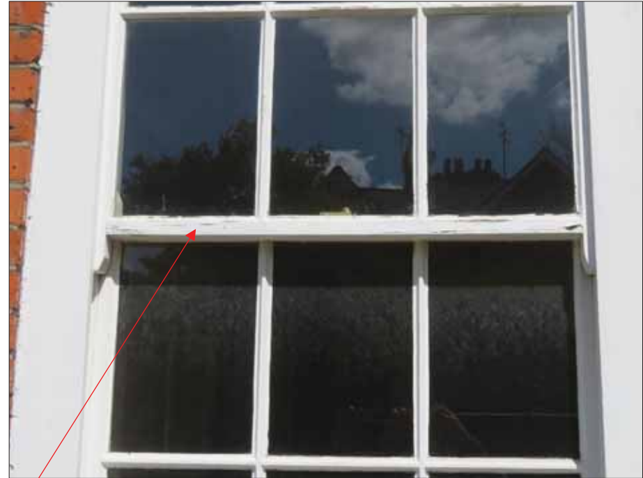
Images 47 & 48: Examples of Decay & Failed Decoration of Sash Windows of the Front Elevation.
