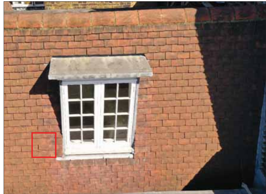
Images 2 & 3: Roof 1 - Front Pitch Showing Handful of Slipped Tiles.
