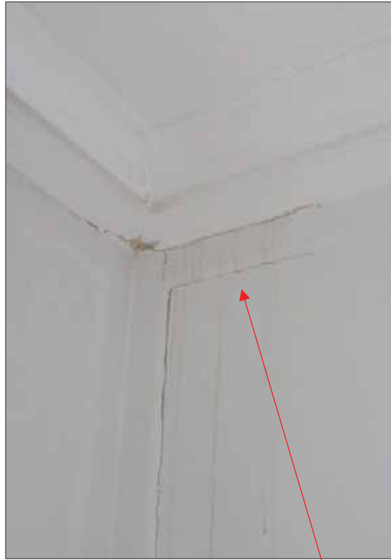
Images 29 – 31: Lead Downpipe to Front Elevation, Corresponding Water Damage Internally & Blockage at its Head.
