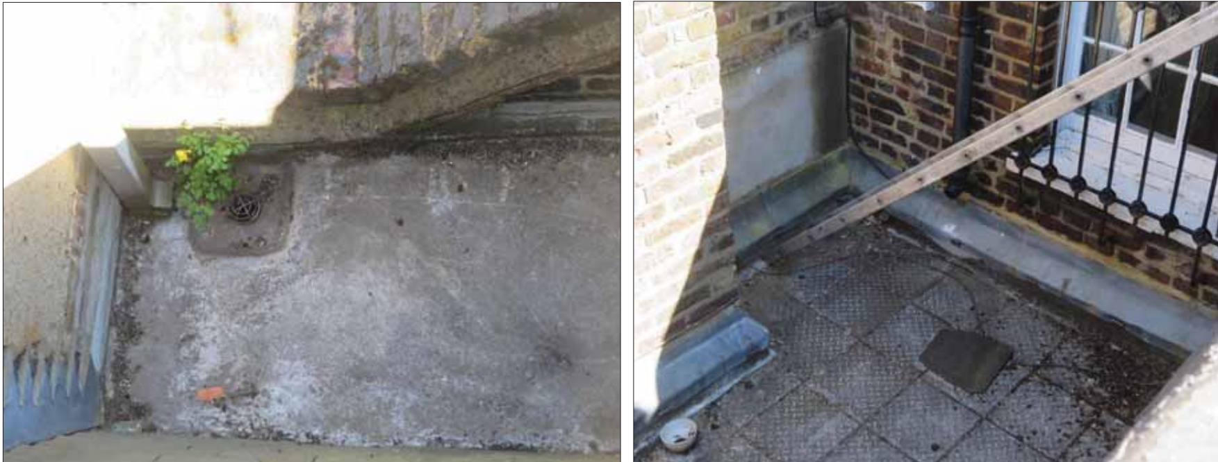
Images 10 & 11: Flat Roof 4 to the West & East, Respectively.
