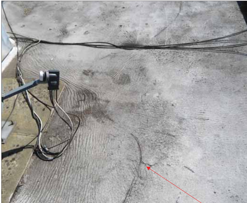
Images 6 & 7: Rippling/Cracking to Roofs 2 & 3, Respectively.
