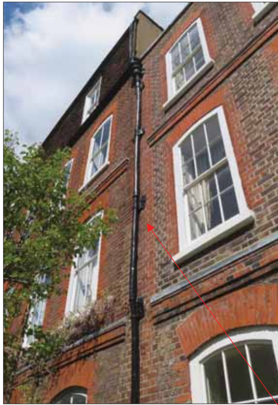
Images 29 – 31: Lead Downpipe to Front Elevation, Corresponding Water Damage Internally & Blockage at its Head.
