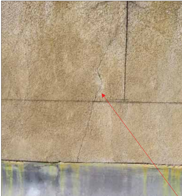
Images 35 & 36: Cracking Render to Western Party Wall at High Level.
