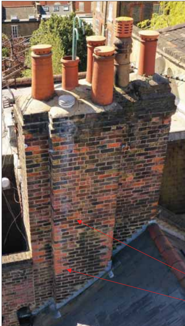
Images 22 & 23: Stacks 1 & 2, Respectively. Note the Spalling Brickwork.
