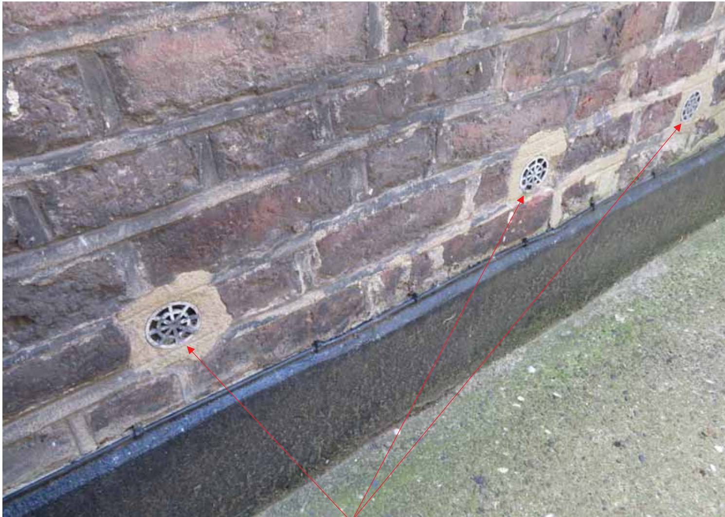
Image 40: Doulton Tubes to the Front Elevation.
