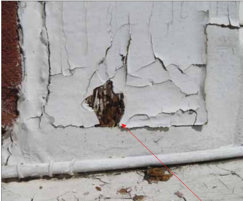
Images 47 & 48: Examples of Decay & Failed Decoration of Sash Windows of the Front Elevation.
