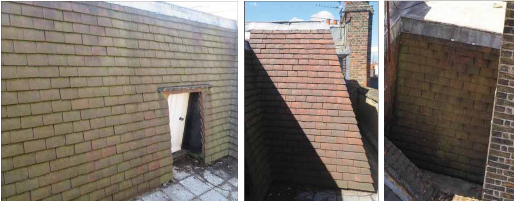
Image 4 -5: Rear Pitches of Roof 1 In Generally Good Condition.
