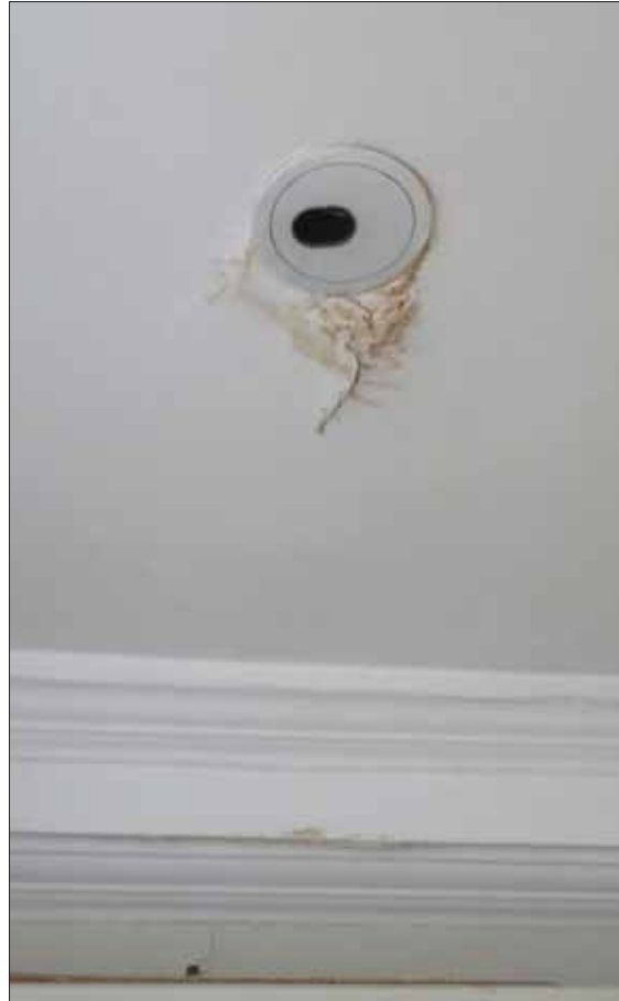
Images 51 – 53: Example Evidence of Plumbing Leaks.
