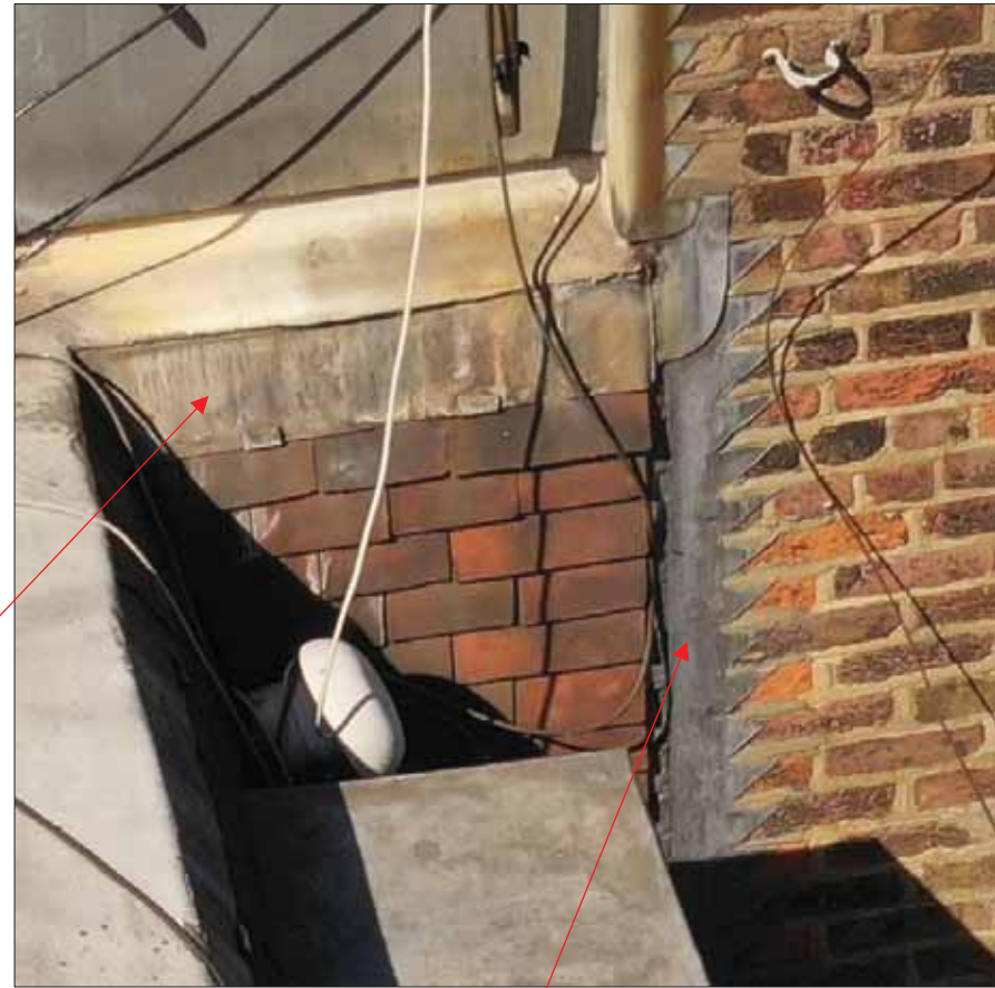
Images 17 & 18: Example Areas of Older Leadwork to the East Party Wall & Top of the Mansard, Note the Newer Leadwork to Stack 1 Adjacent.
