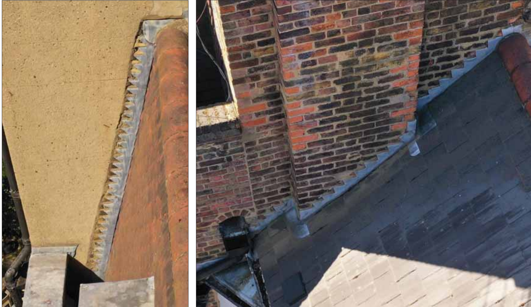
Images 19 & 20: Newer Leadwork Elements to the West Party Wall & Roof 5.
