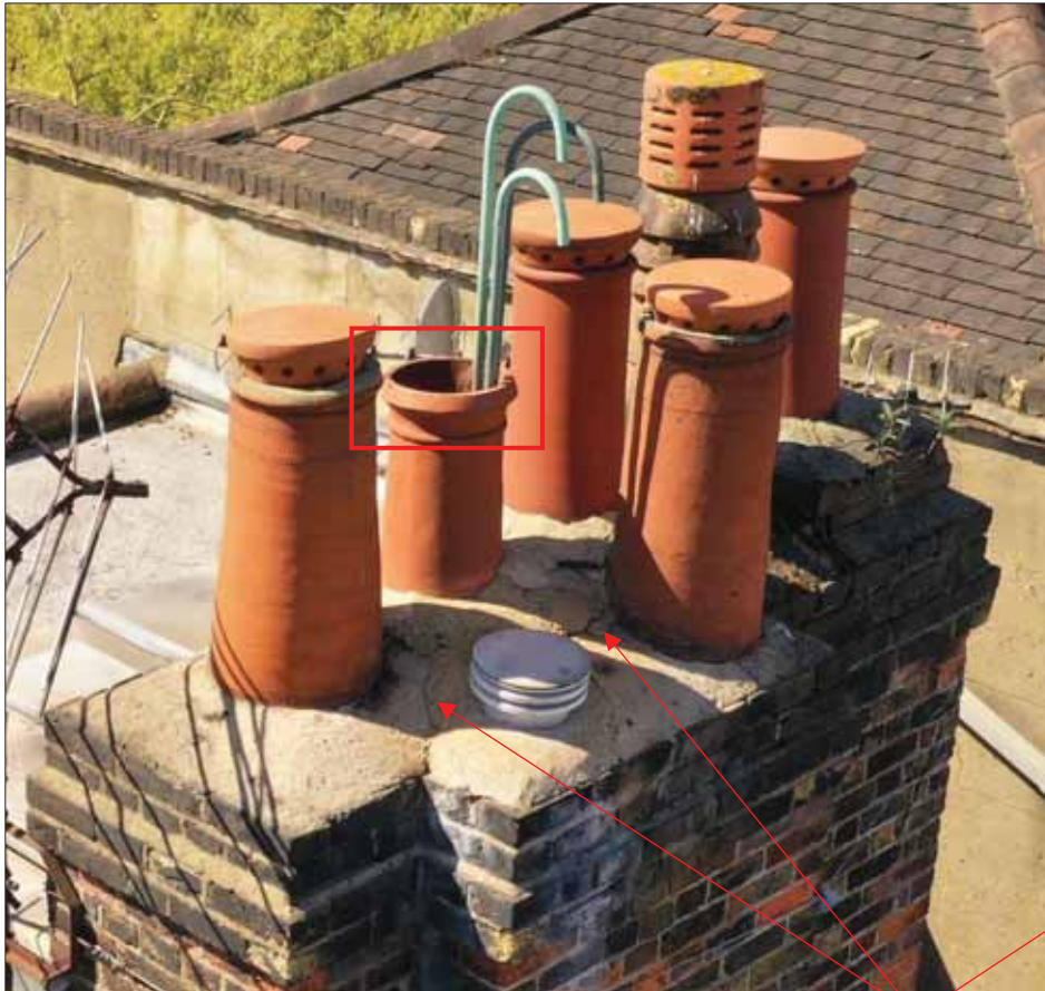
Images 24 & 25: Showing Cracking to Flaunching & Two Pots Without Cowls.
