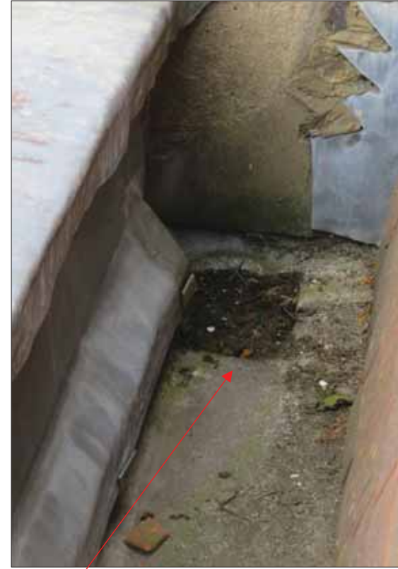
Images 29 – 31: Lead Downpipe to Front Elevation, Corresponding Water Damage Internally & Blockage at its Head.
