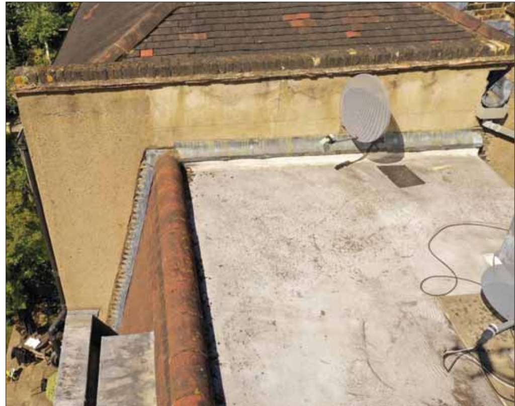
Images 35 & 36: Cracking Render to Western Party Wall at High Level.
