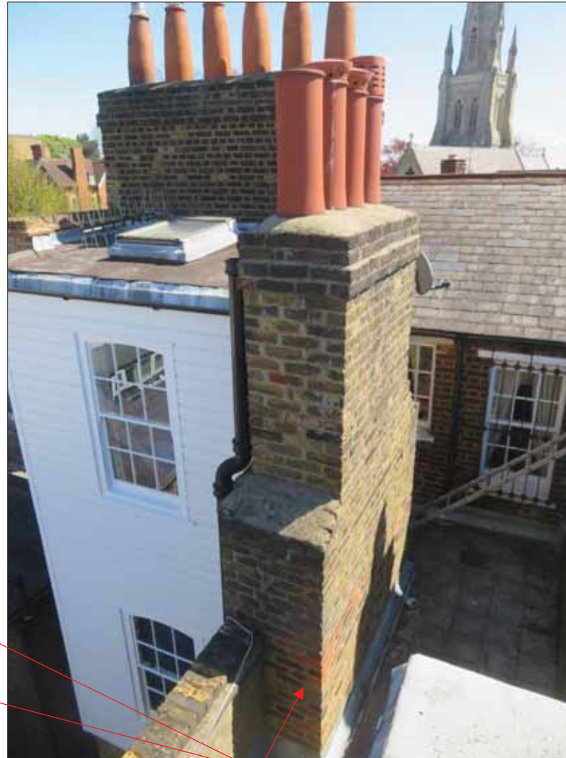
Images 22 & 23: Stacks 1 & 2, Respectively. Note the Spalling Brickwork.
