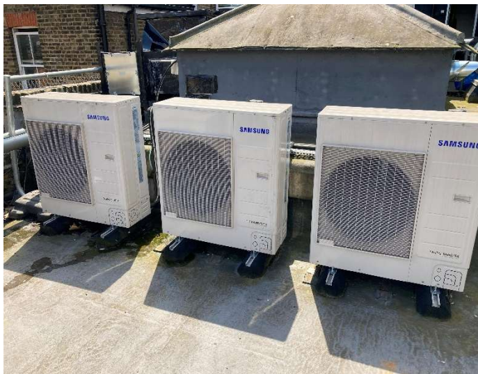
Figure 4: Replacement air conditioning condenser units
