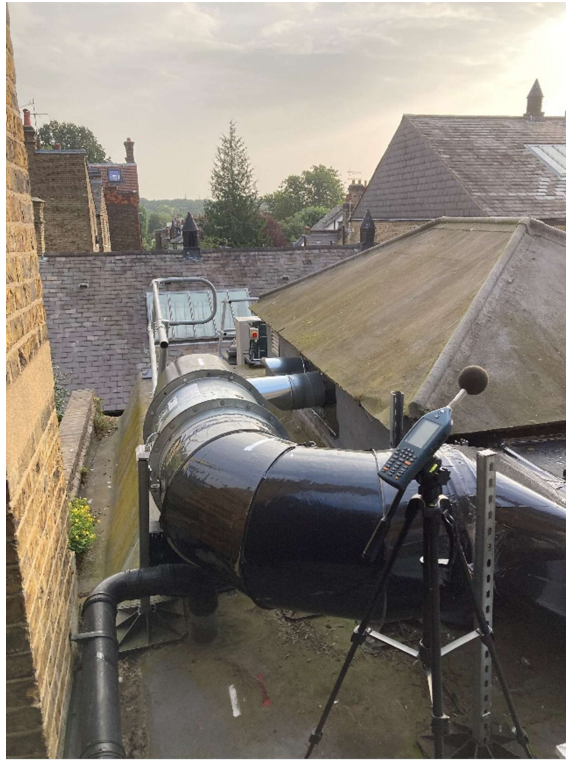
Figure 3: Modified kitchen supply ductwork
