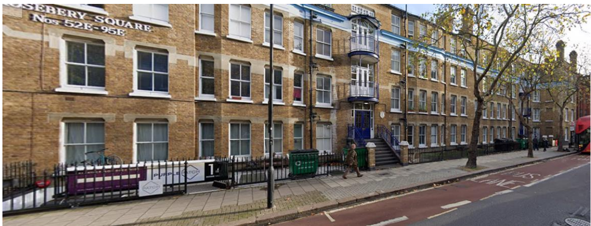
Photo 4: Front elevation of Rosebery Square showing existing lightwells
