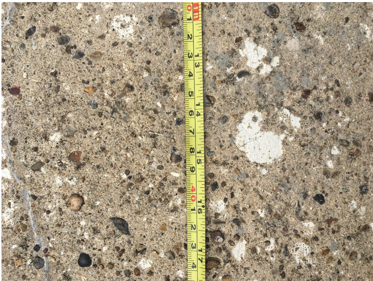
Cleaned surface of terrace showing aggregate and binder
