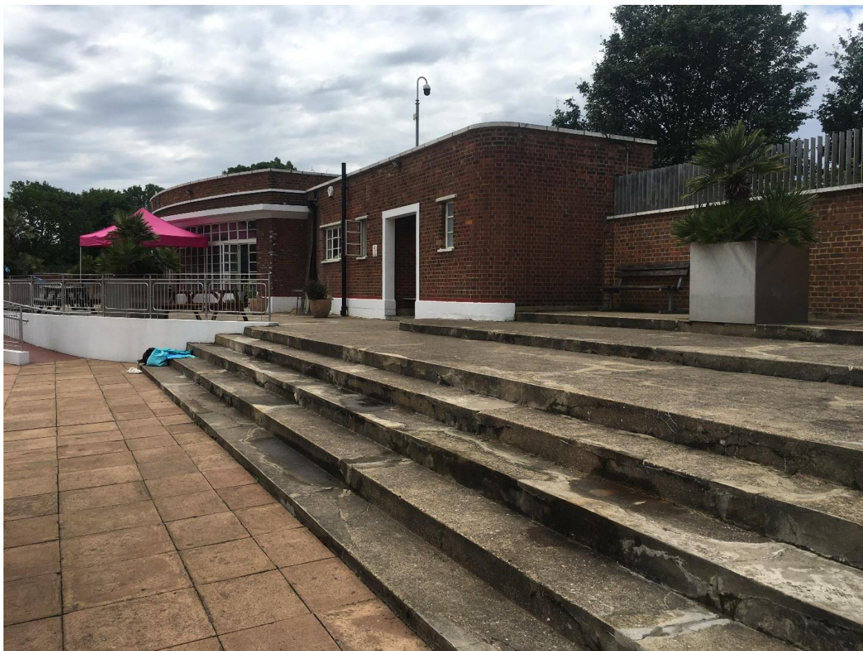
North-west terrace and steps with café / gymnasium to left
