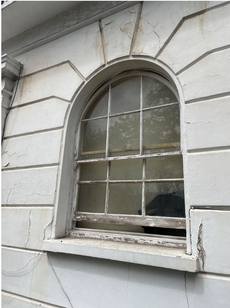
Figure 8: External view of the timber sash window in the sitting room at ground floor level
