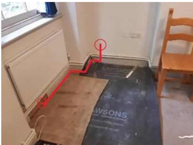
Figure 2 – Internal basement flat route (existing heating pipes on the wall to be lowered under the new gas pipe)
