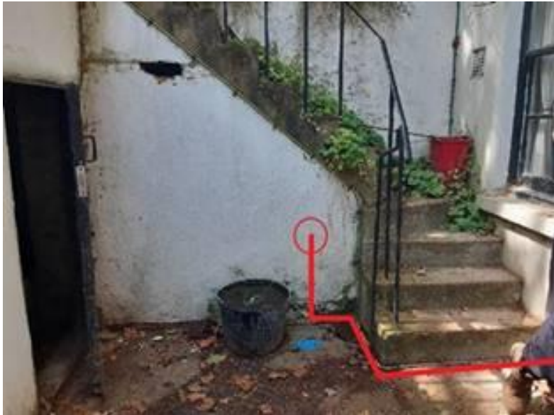
Figure 3 – Lightwell at the front of House 47 (External route from the basement flat to the gas meter.) By looking through an existing void in the wall below the steps in the lightwell we
