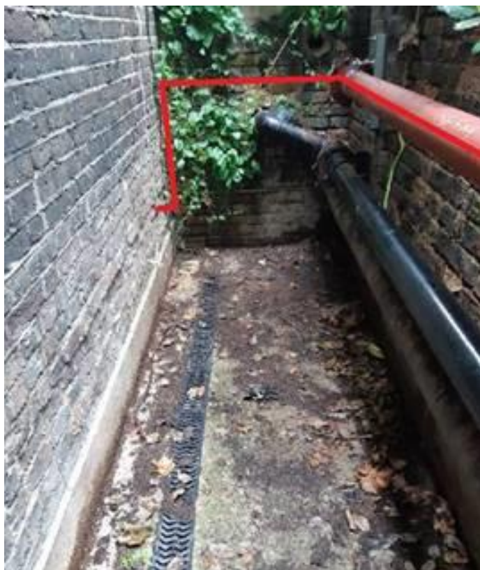
Figure 1 – External lightwell running along the side of House 47
