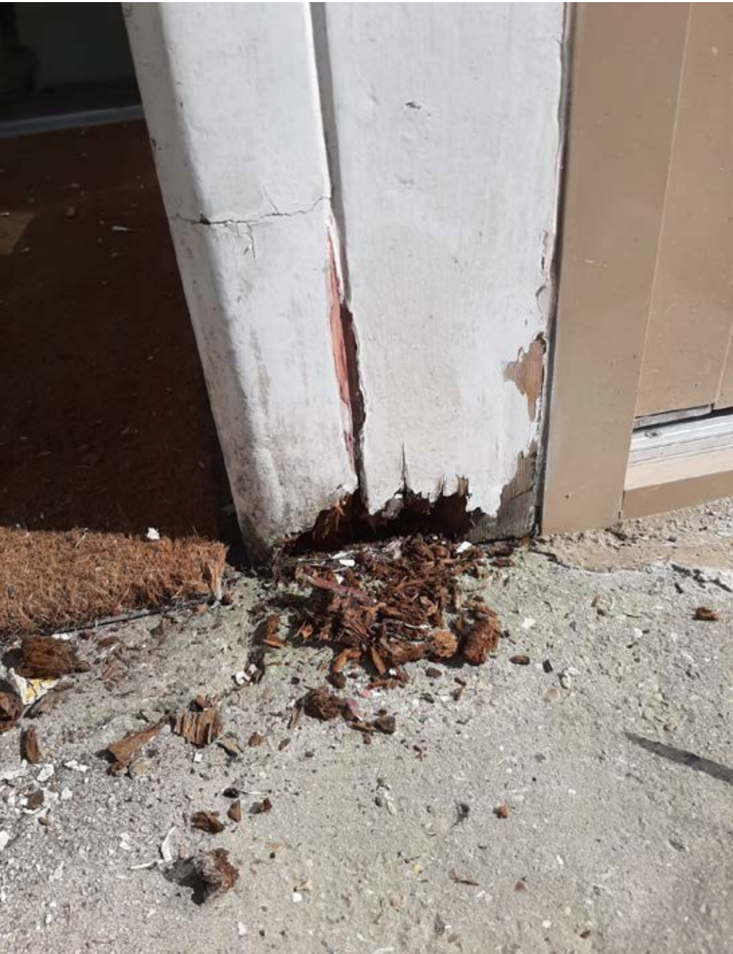
Images of termite damage to the existing wooden doors and windows
