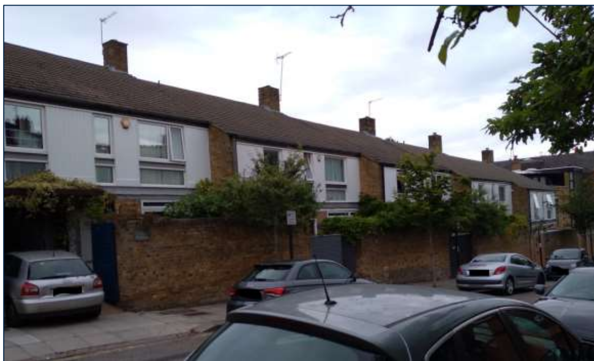
Figure 3: Front gardens to Nos. 31-39 Rudall Crescent
