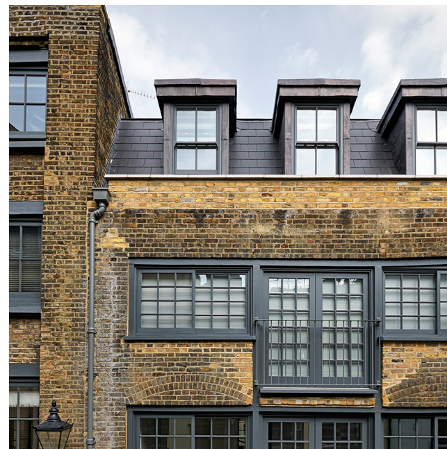
Fig 10. Obscured Glass Balustrades to Terraces. Fig 11. Yellow Stock Brickwork, slated mansard & lead dormers.
