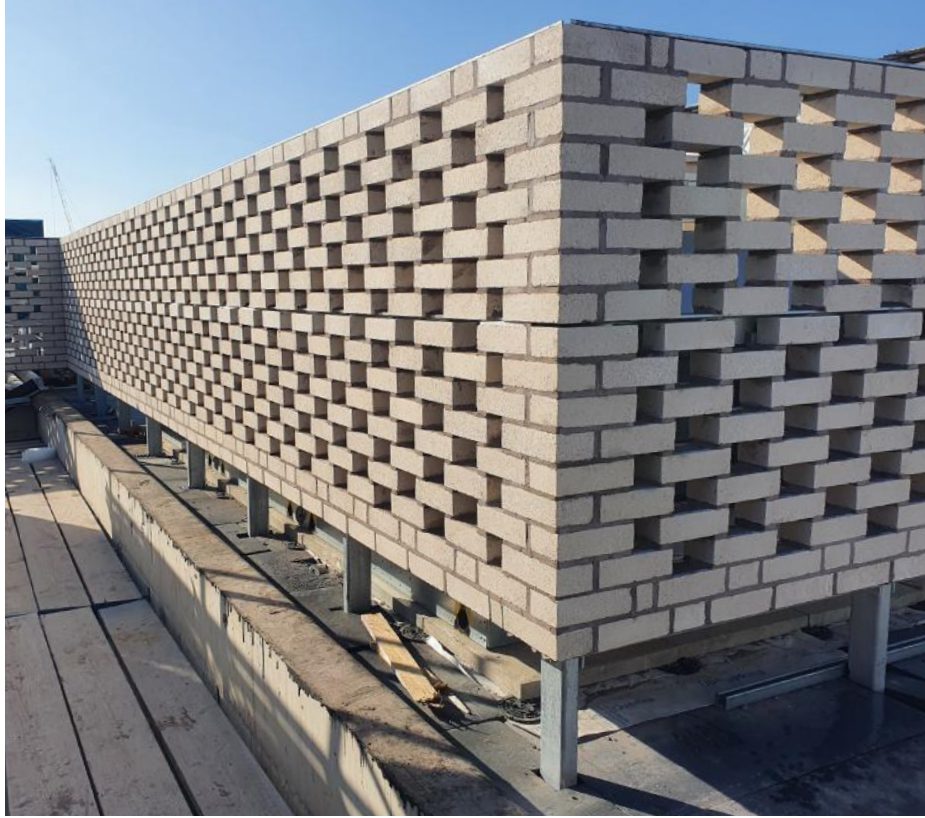
Enenhall Caselton White concrete brick (to match main elevations and discharged separately) mounted on a galvanised structural frame
