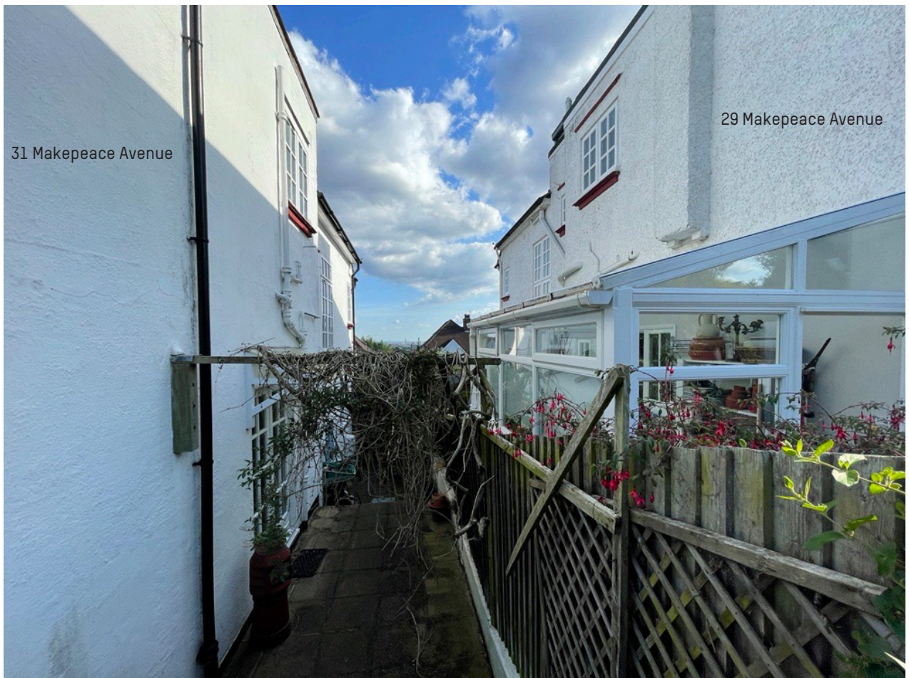
Existing View - Side Passage of 31 Makepeace Avenue
