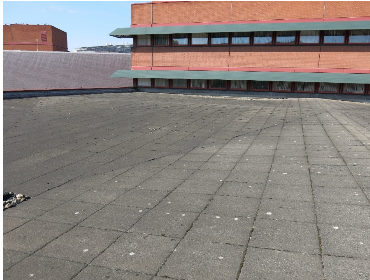
Plate 5: Overall context photograph of roof level 4 – showing precast concrete slabs and falls to existing gullies
