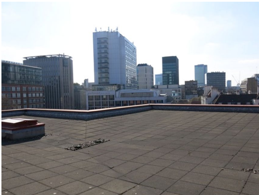
Plate 4: The lower roof, Level 4, looking west towards the Pullman Hotel - shows the levels and falls to the rainwater outlets.
