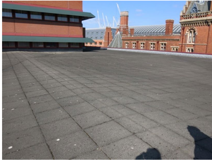
Plate 3: The lower flat roof, Level 4, looking north-east toward St Pancras Station – shows the levels and falls to the rainwater outlets.
