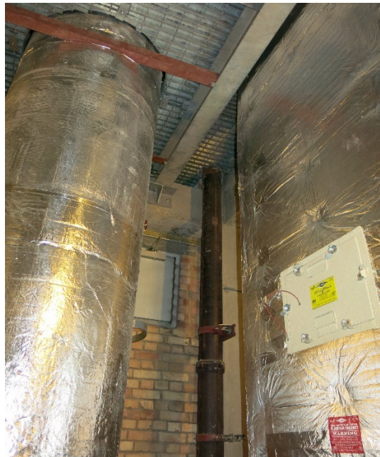
Plate 7: Service intermediate floor service riser- pipework to be installed against corner of wall leading to basement plant room
