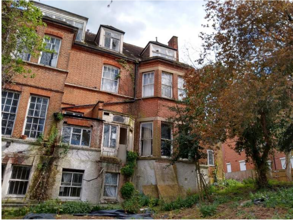
Photo 8: shows building B1 which is dilapidated. Although currently lived in.
