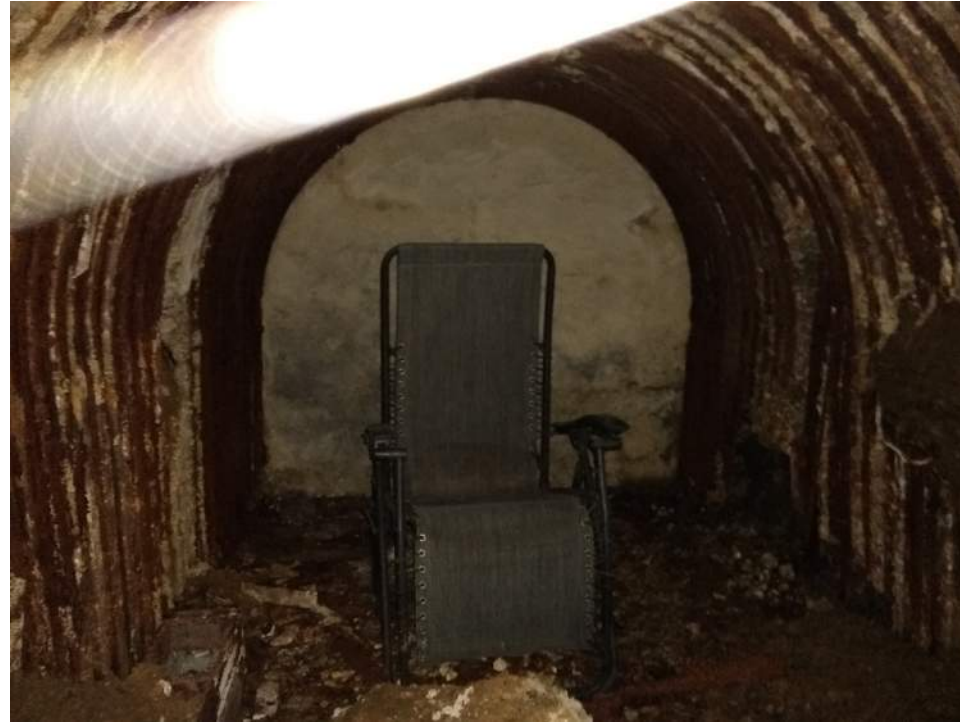
Photo 9: shows the interior of the bomb shelter, building B2
