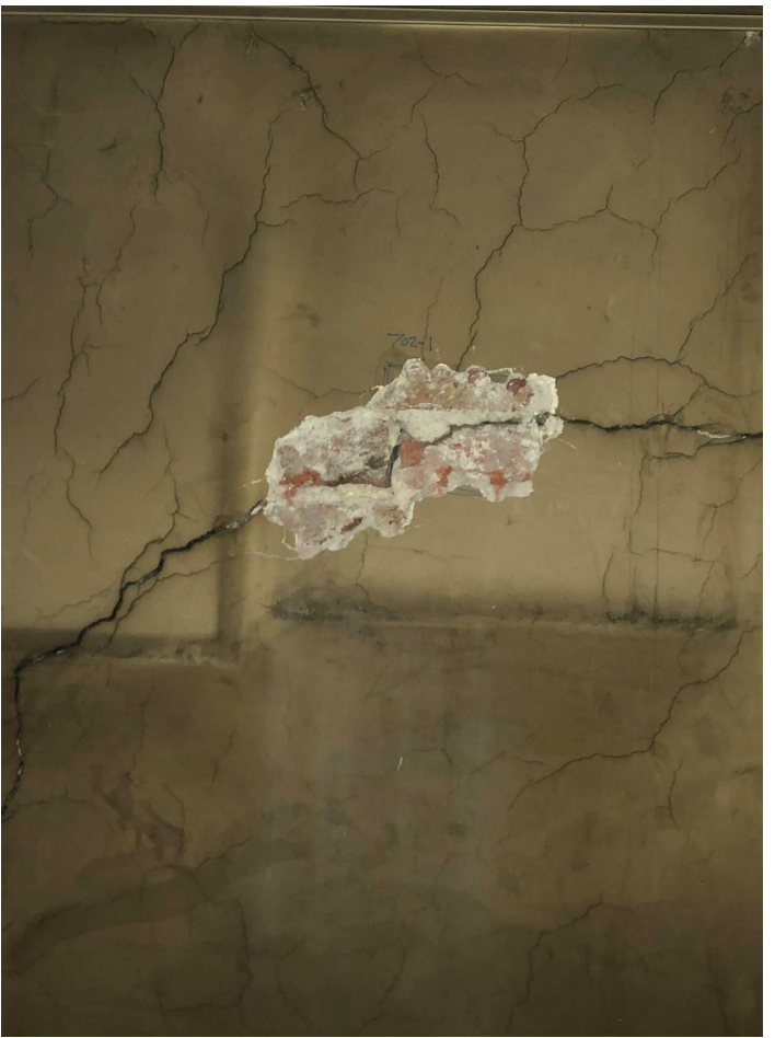
Existing Metal Floor, Timber Access Stair to be removed. Cracks in historic lime plaster to be repaired by plaster specialist in lime.
