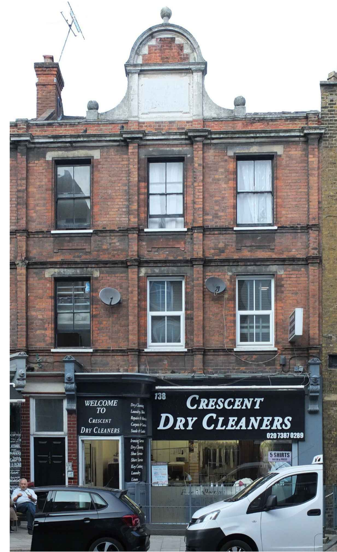
02 Existing Photo Elevation
