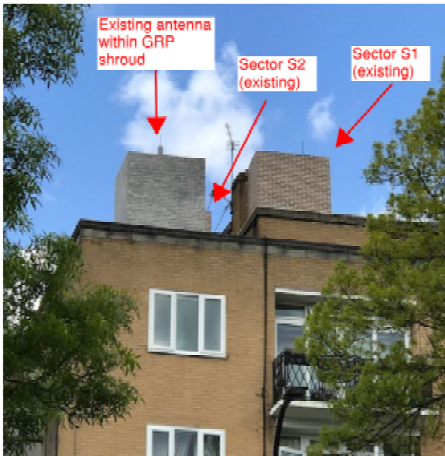
Image 5 – view of Portland Court from east
