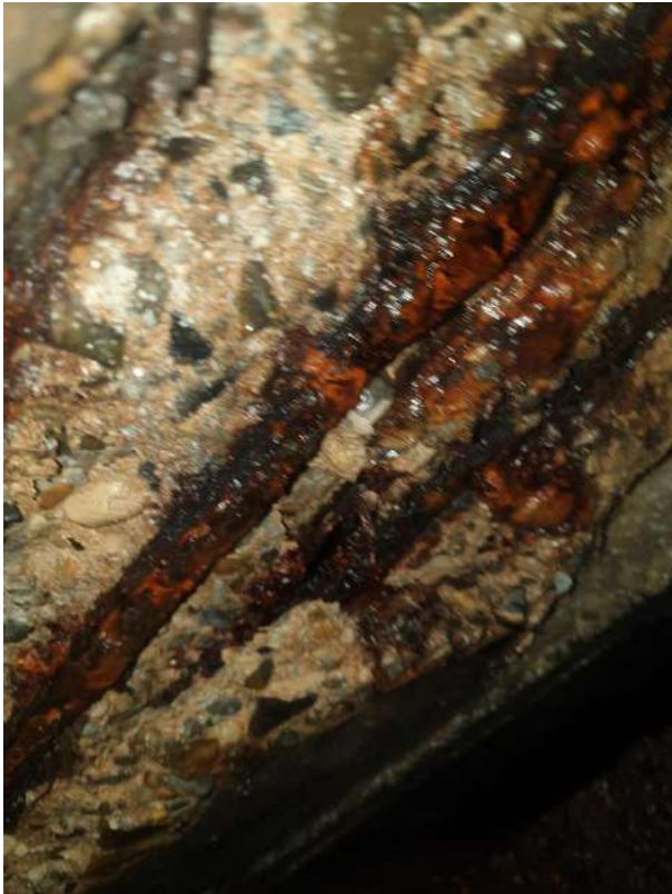
MH2 LOOKING TOWARDS MH1 – CORROSION BEGINS 2 METRES IN FROM MH2 TOWARD MH1
