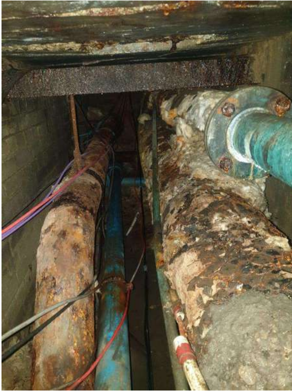
MH2 LOOKING TOWARDS MH1 – CORROSION BEGINS 2 METRES IN FROM MH2 TOWARD MH1
