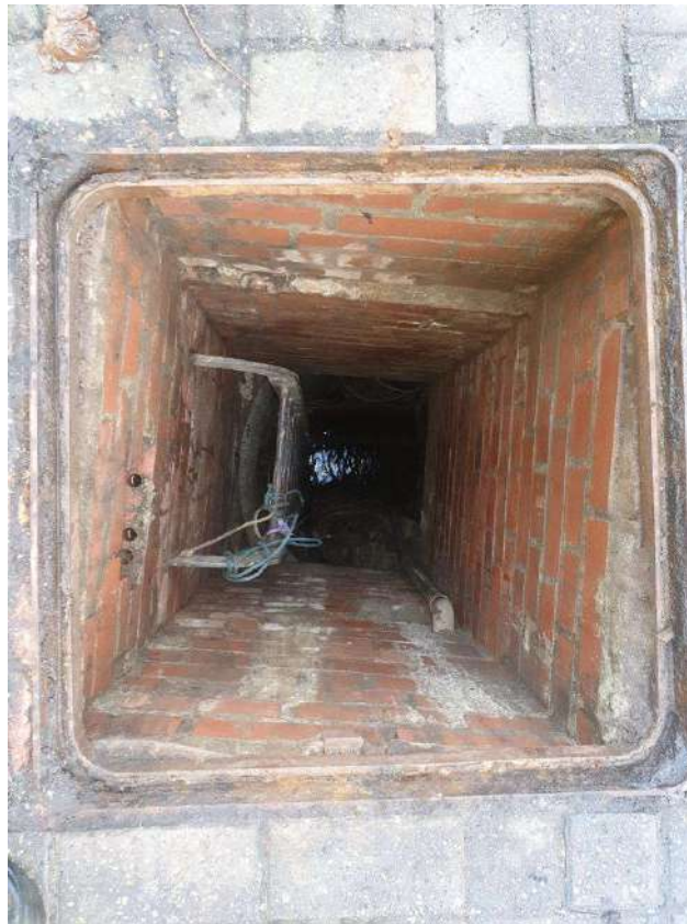
MH1 AT SURFACE
