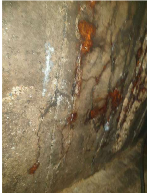
MH2 LOOKING TOWARDS MH1 – CORROSION BEGINS 2 METRES IN FROM MH2 TOWARD MH1
