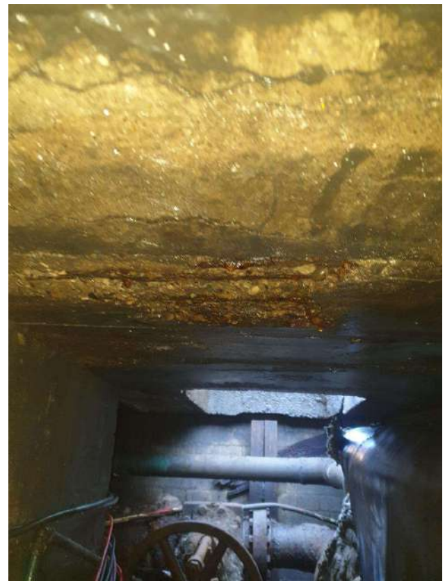
CORROSION BEGINS 2 METRES FROM MH2 TOWARD MH3
