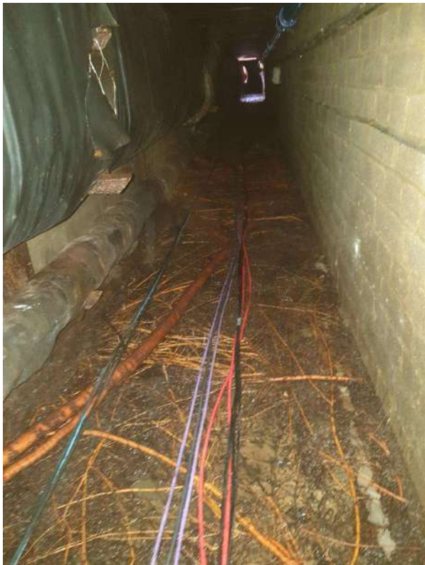
MH4 TOWARDS MH5 – SMALL TREE ROOTS, ENTIRE LENGTH OF RUN
