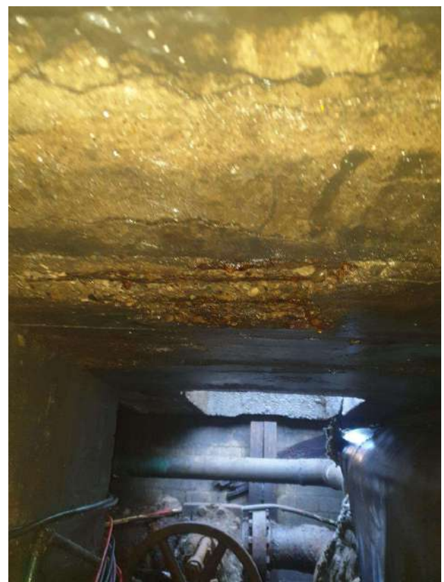
CORROSION BEGINS 2 METRES FROM MH2 TOWARD MH3
