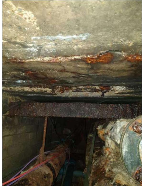
MH2 LOOKING TOWARDS MH1 – CORROSION BEGINS 2 METRES IN FROM MH2 TOWARD MH1
