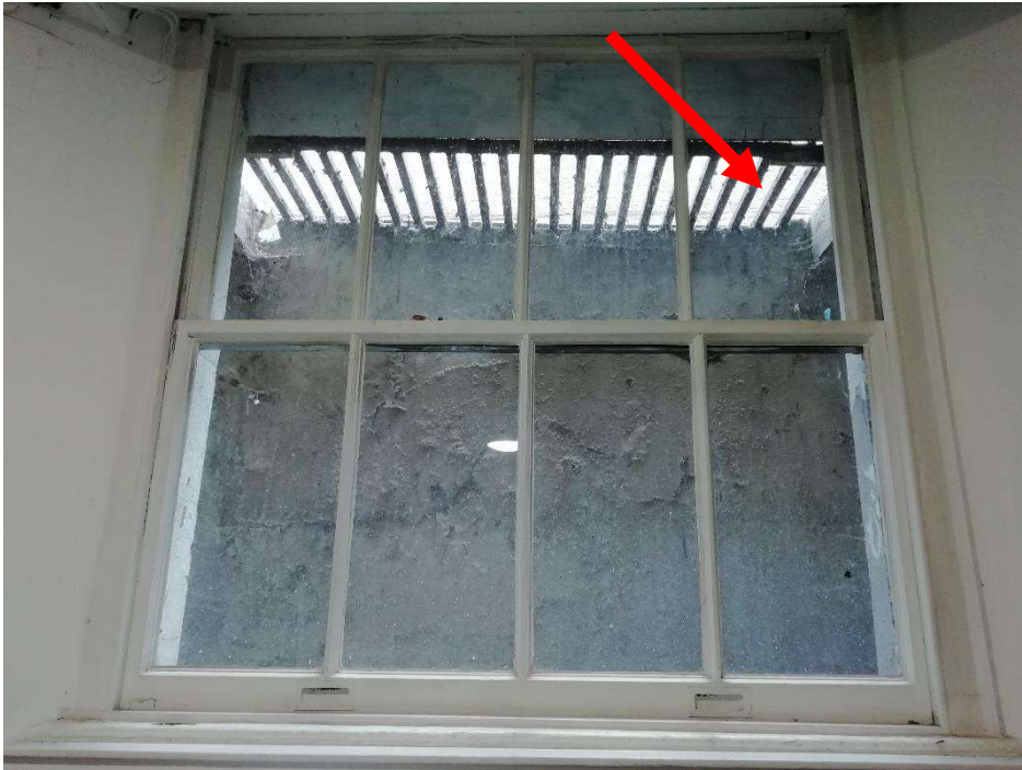
Figure 8: Basement window. One pane will be replaced with Perspex, red arrow.
