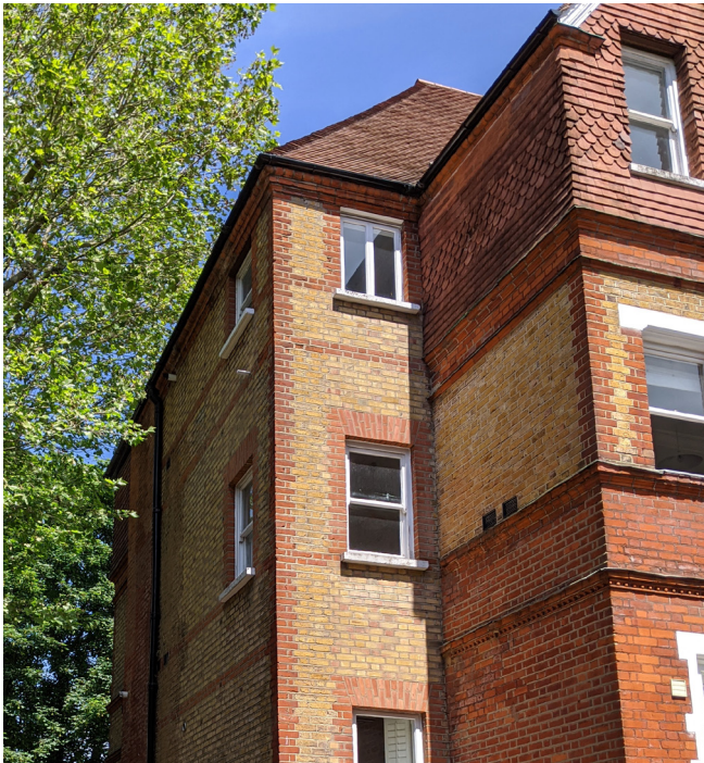
Side View with Existing Flues/Vents
