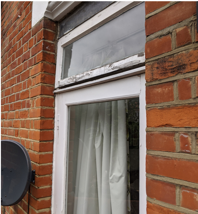
Existing Condition of Balcony Doors
