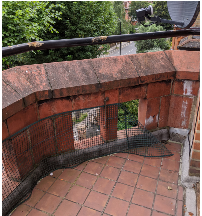
Existing Condition of Balcony with Mesh for Protection from Falling
