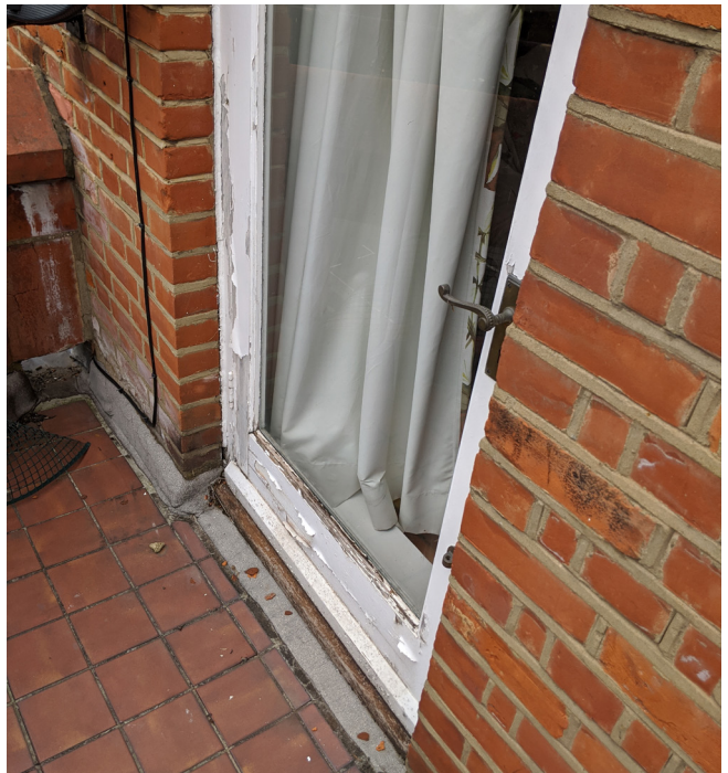
Existing Condition of Balcony Doors
