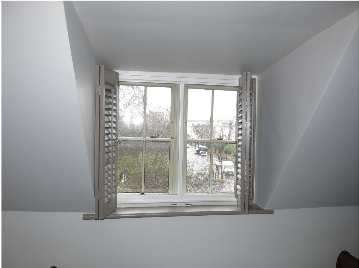
Figure 13 – Internal view of two timber sash windows with bedroom 3 on the second-floor level
