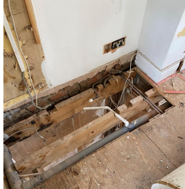
Plywood floor taken up to reveal notched joists
