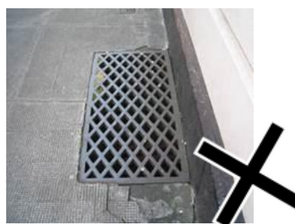
Grille – not acceptable
