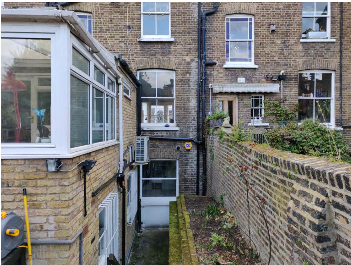
[Fig. 05] Side View of Existing Conservatory Showing Lower Ground Floor Level
