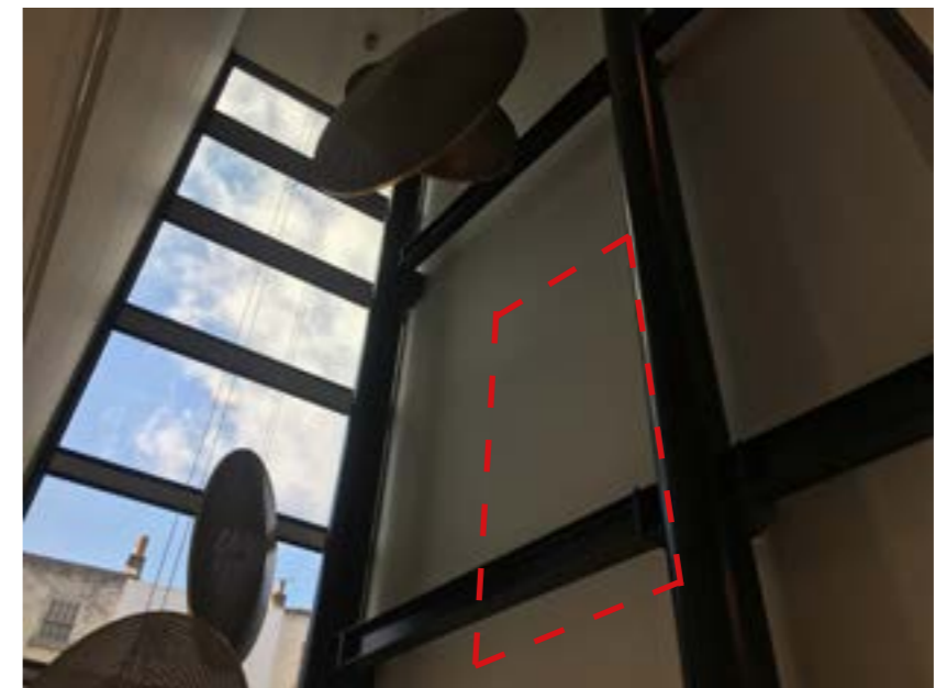
Existing view within Kings Cross Bridge
