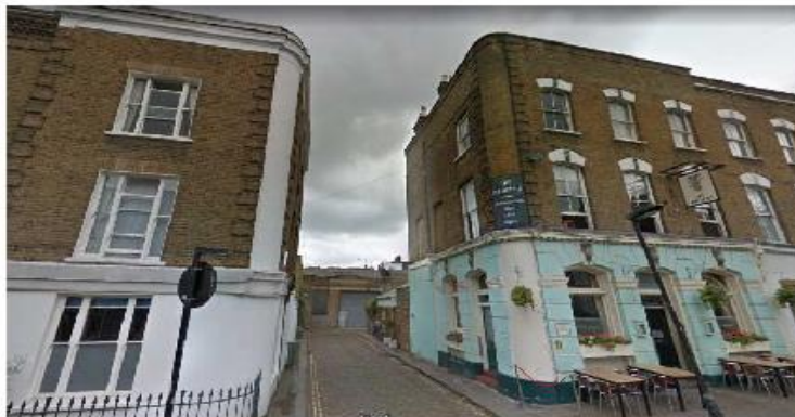
3) Long view of site down Railey Mews, The Pineapple (Grade II Listed pub) in foreground
