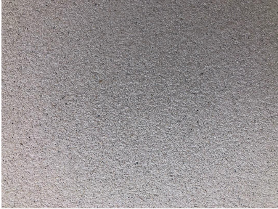
Photograph 7: Close-up detail of surface finish to GRC panels
