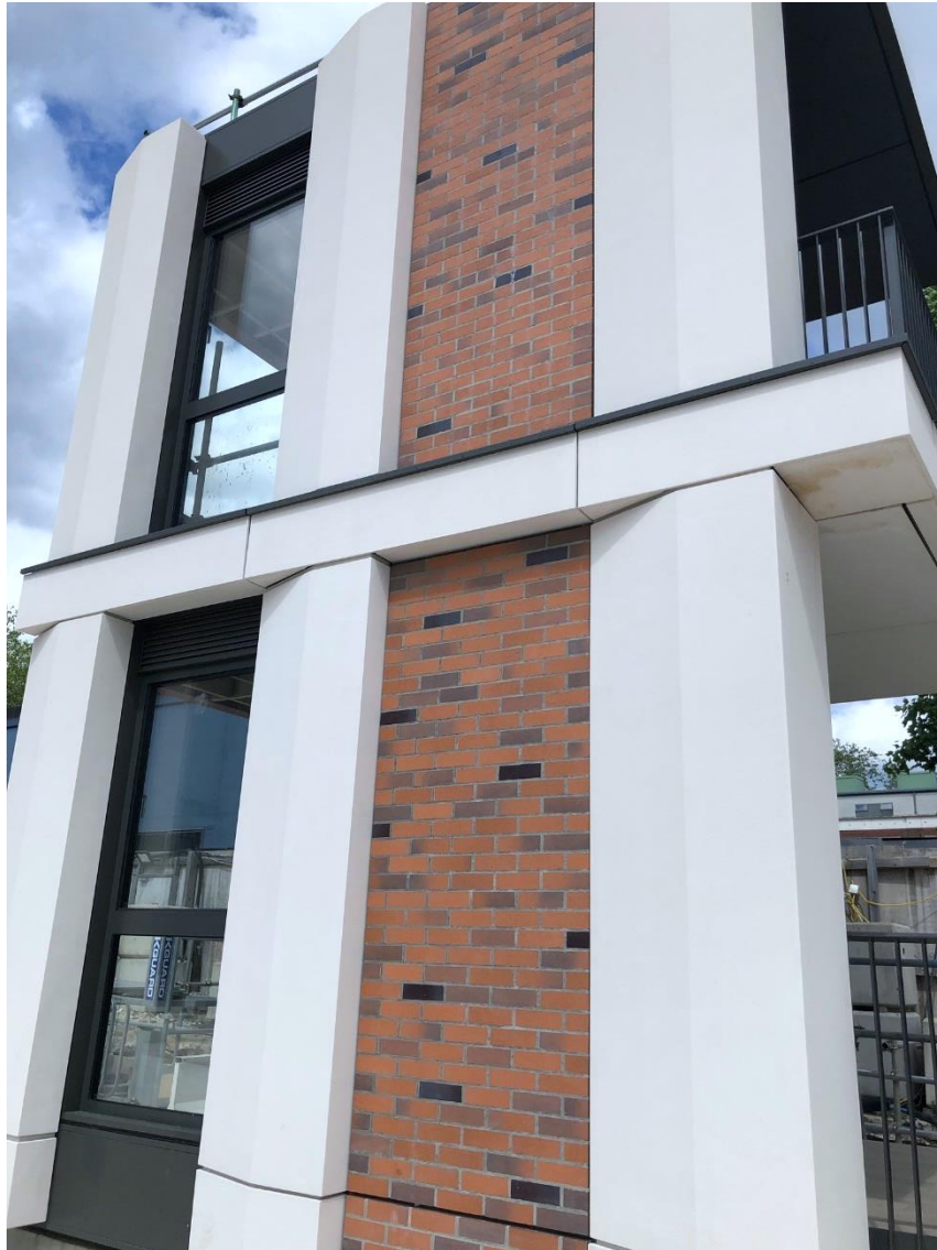
Photograph 6: Fully-scaled sample panel with GRC panels and detailing
