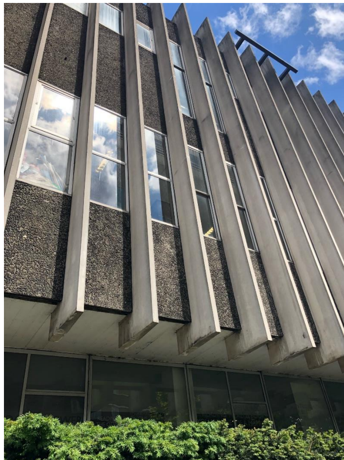
Photographs 3 & 4: Swiss Cottage Library – external façade details; concrete fins, pre-cast basalt concrete aggregate panels, board-marked concrete soffit, aluminium windows and ashlar Portland stone base.
