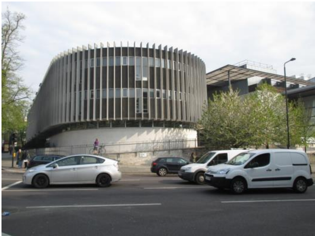
Photograph 2: Swiss Cottage Library – raised south end with vertical concrete fins, pre-cast concrete aggregate spandrel panels, aluminium strip windows and Portland stone plinth.
