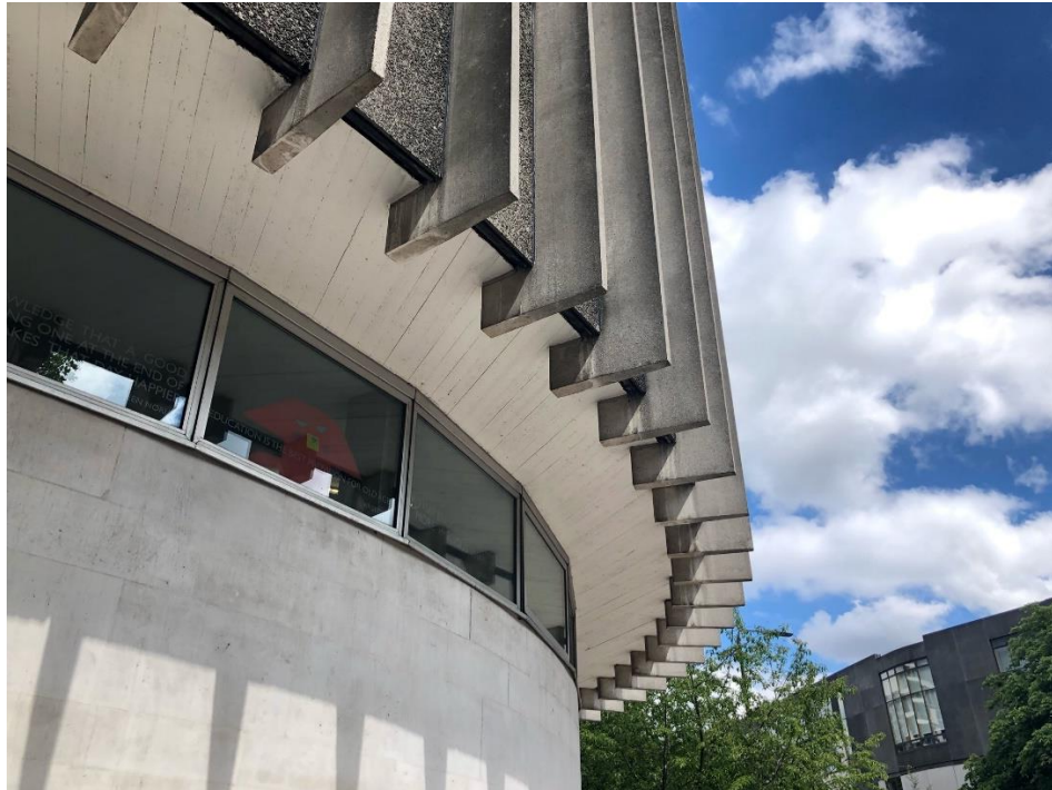
Photographs 3 & 4: Swiss Cottage Library – external façade details; concrete fins, pre-cast basalt concrete aggregate panels, board-marked concrete soffit, aluminium windows and ashlar Portland stone base.
