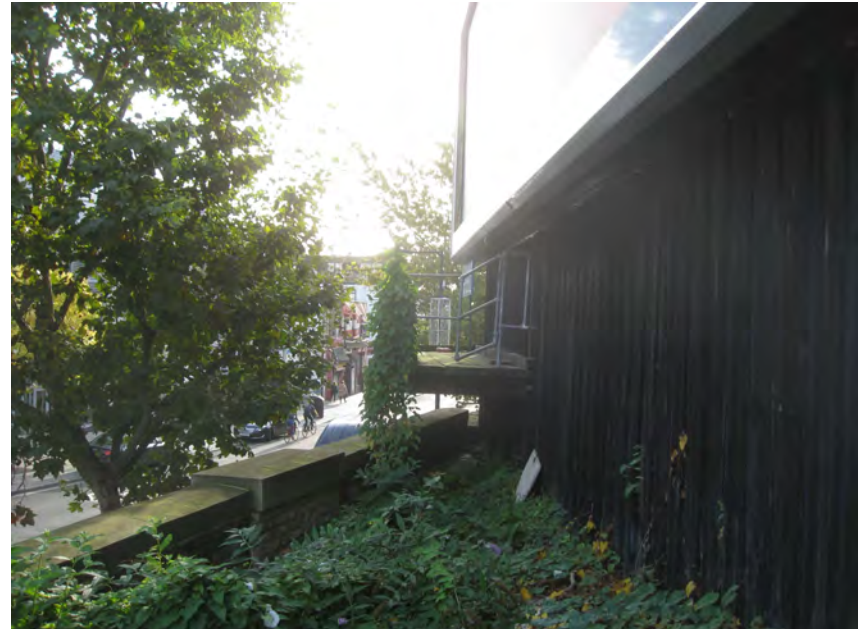
Retaining wall to north end of site – east corner
