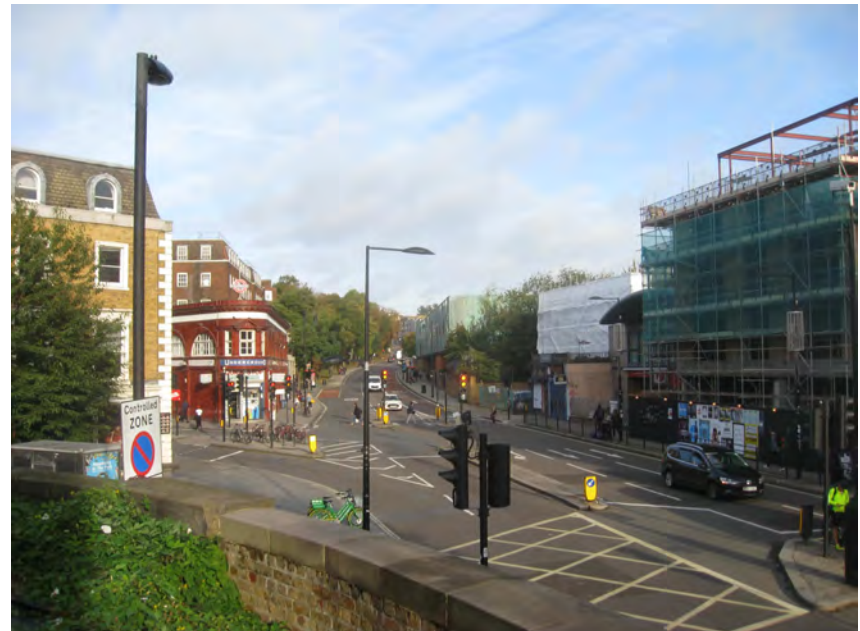
Retaining wall to north end of site – north west
