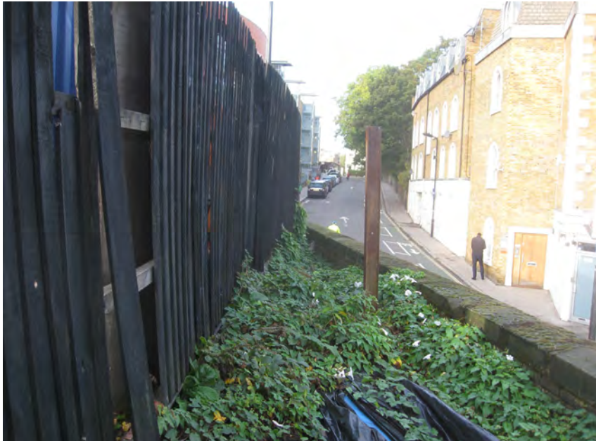
Retaining wall to north end of site - south west
