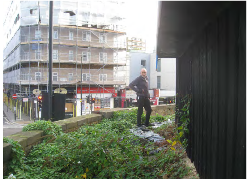
Retaining wall to north end of site - north
