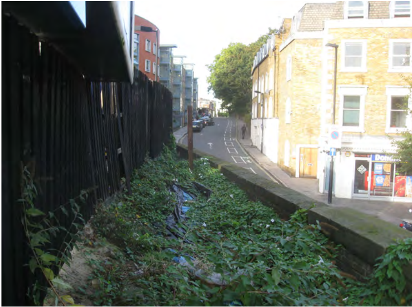
Retaining wall to north end of site – west
