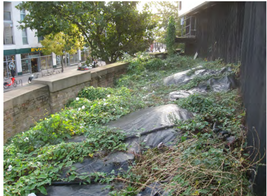
Retaining wall to north end of site - east
