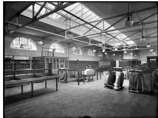
Figure 11: Stanmore sorting office in an undated photograph. This building also had an overseer's window at one end and similar Diocletian windows to those seen at Kentish Town.
