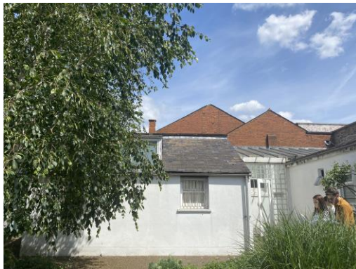
Figure 5: Original WC block to the rear of the site.
