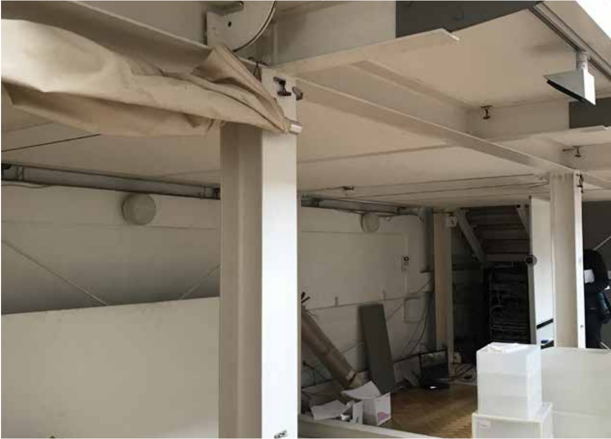
3. Existing mezzanine structures with dark, low quality storage space below
