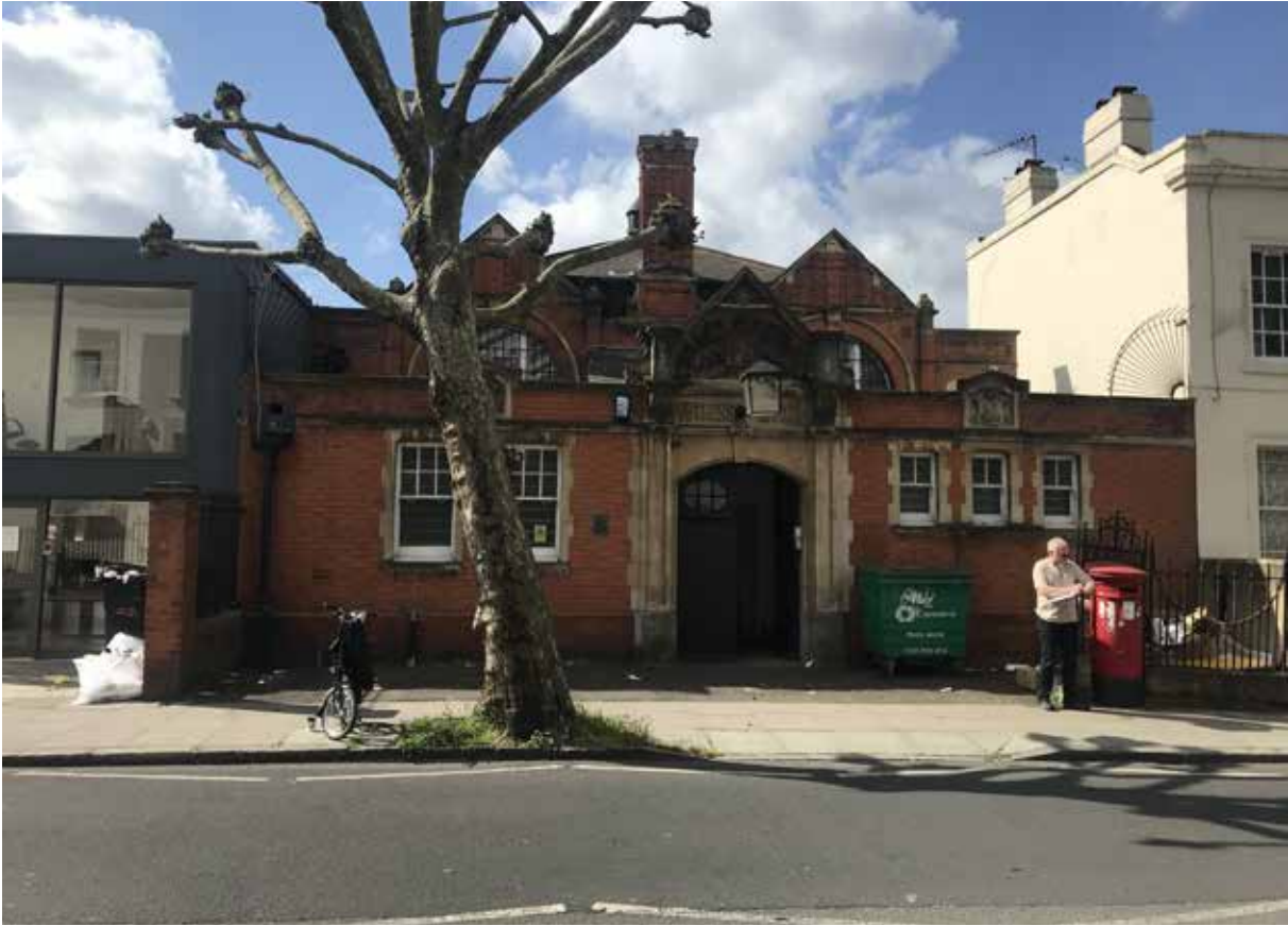
1. View of existing entrance with bin and rubbish dumped behind railing
