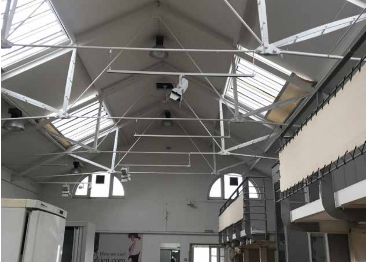
5. Existing roof trusses and rooflights
