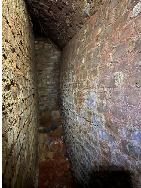
Photo 2: Severe bulge in vault wall
