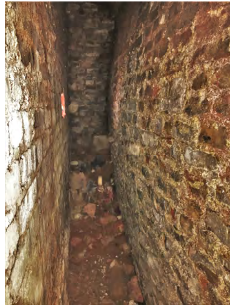
Photo 3: Severe bulge in vault wall
