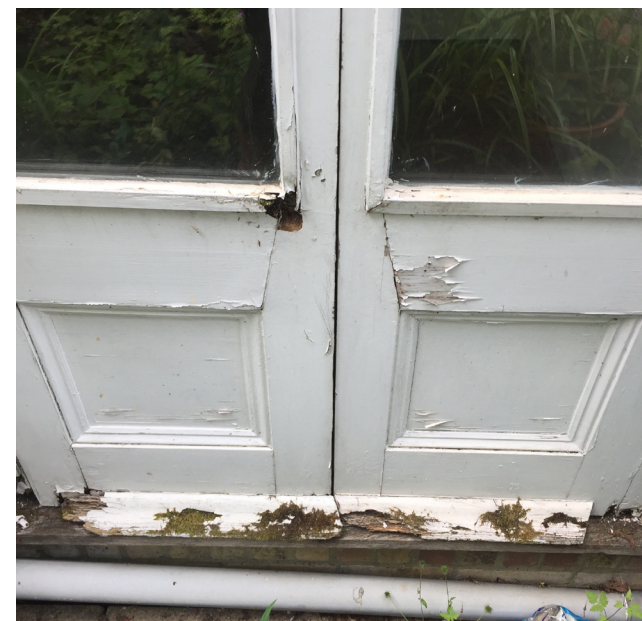
Figure 6. Rotten door frame at 75 Belsize Lane.
