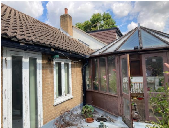
Figure 2: Rear elevation and conservatory from first floor roof terrace
