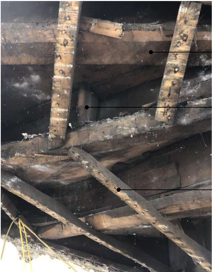
S1.4 Timber beams to suit profile of stair as S1.3 Main stair supporting beam Packing pieces to make up stair riser Lath fixed to timber straights
