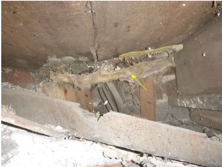
Photograph 7. Visible historic dry rot to the underside of the lower flight of the 1 st to ground floor staircase.
