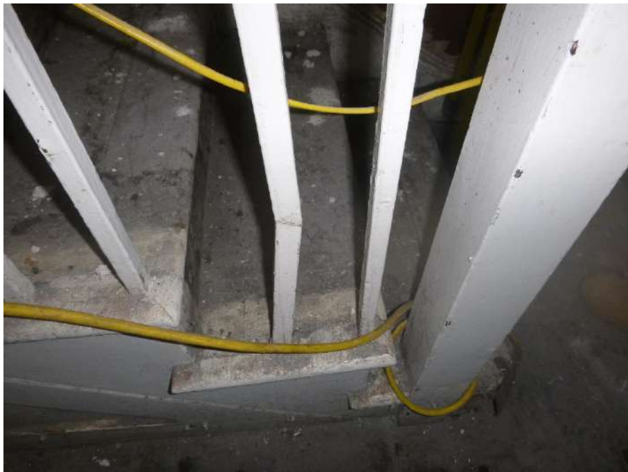
Photograph 6. Broken baluster in the lower flight of 1 st to ground floor staircase.
