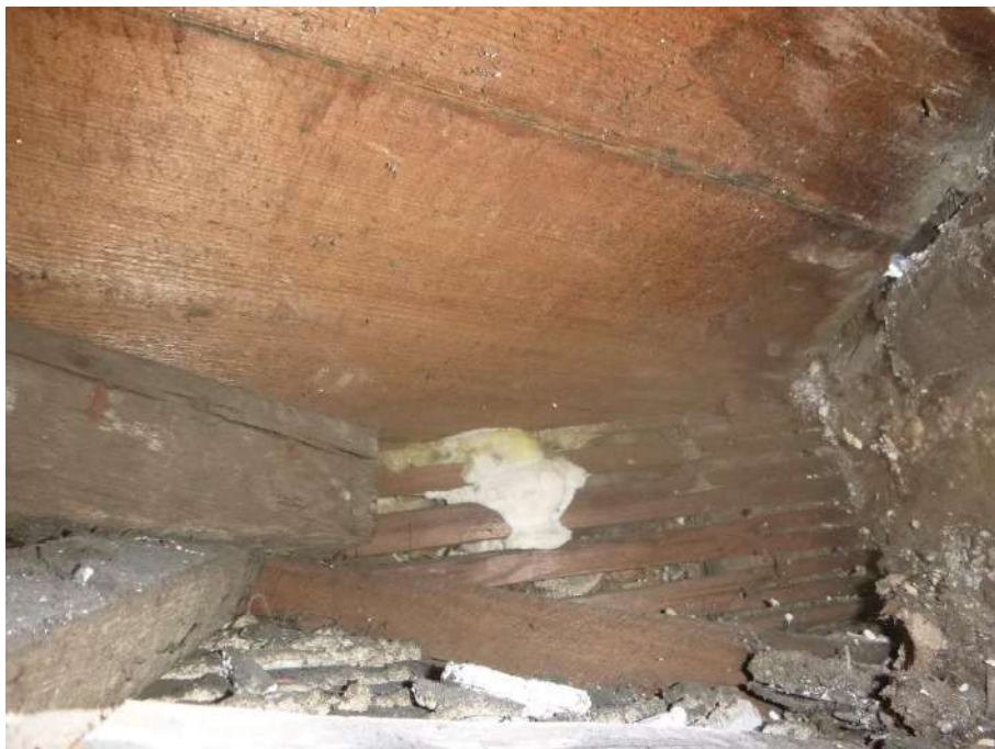
Photograph 2. Visible mycelium on wall laths adjacent to stringer on upper flight of 3 rd to 2 nd floor.
