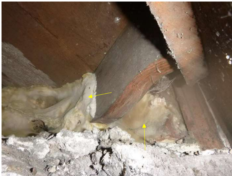
Photograph 4. Historic fungal decay in the upper flight of the 2 nd to 1 st floor staircase.
