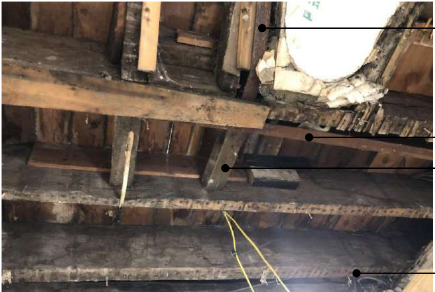
S1.4 Cranked steel RSJ Supporting RSJ (off masonry) Timber blocking (assumed restraint to RSJ) Main timber floor joists running parallel to RSJ. Measured 240mm dp x 50mm wide
