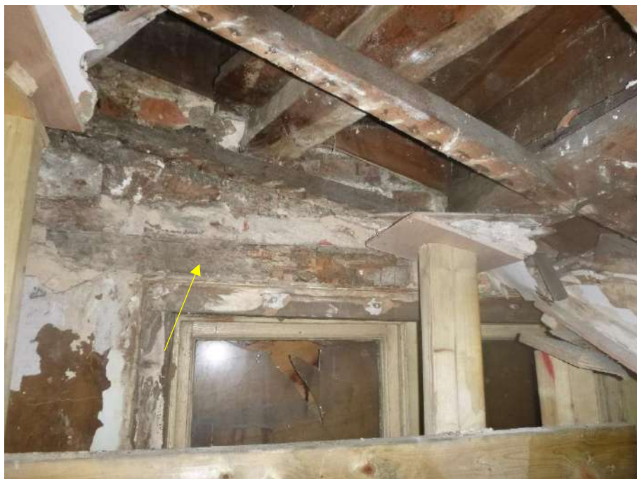
Photograph 10. Lintel between the 2 nd and 1 st floors.
