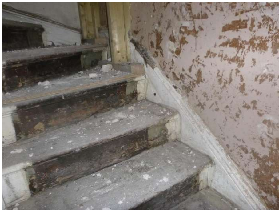
Photograph 8. Lower flight of 1 st to ground floor subject to extensive fungal decay.
