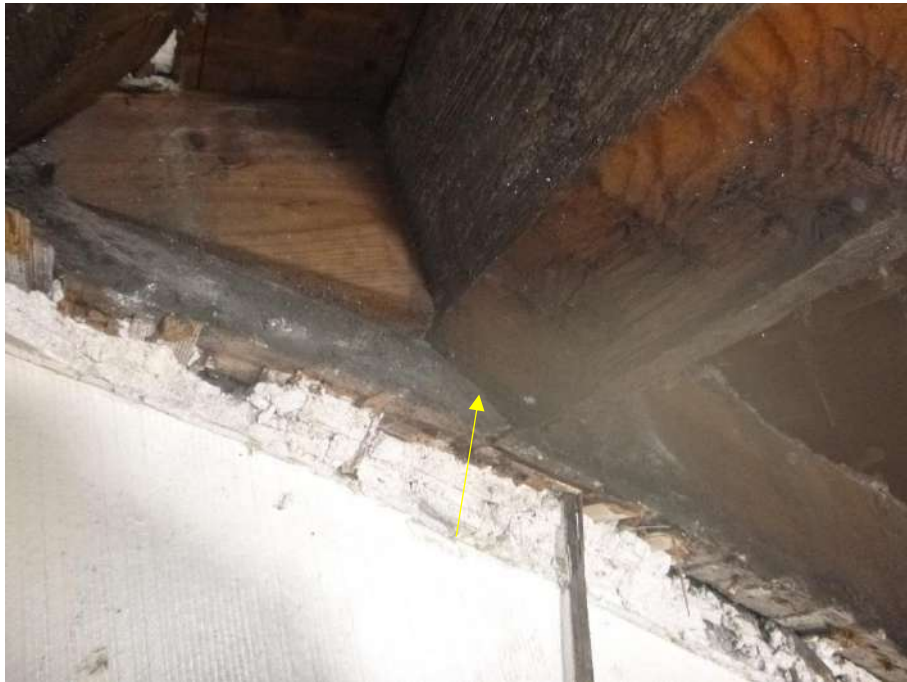
Photograph 5. Fracture in the stringer in the lower flight of the 2 nd to 1 st floor staircase.
