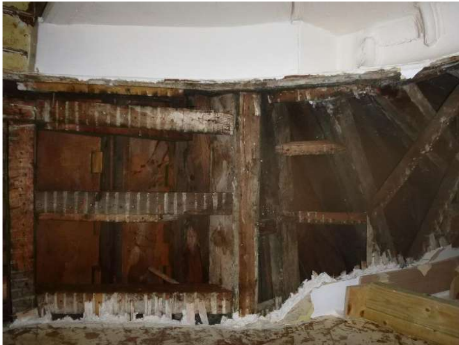
Photograph 1. Underside of upper stair winder from 3 rd to 2 nd floor.
