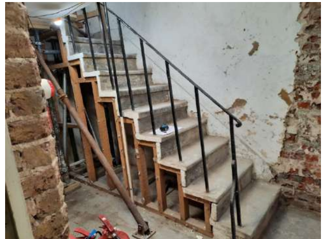
Figure 6. Existing Basement Stair in 48 with metal spindles.
