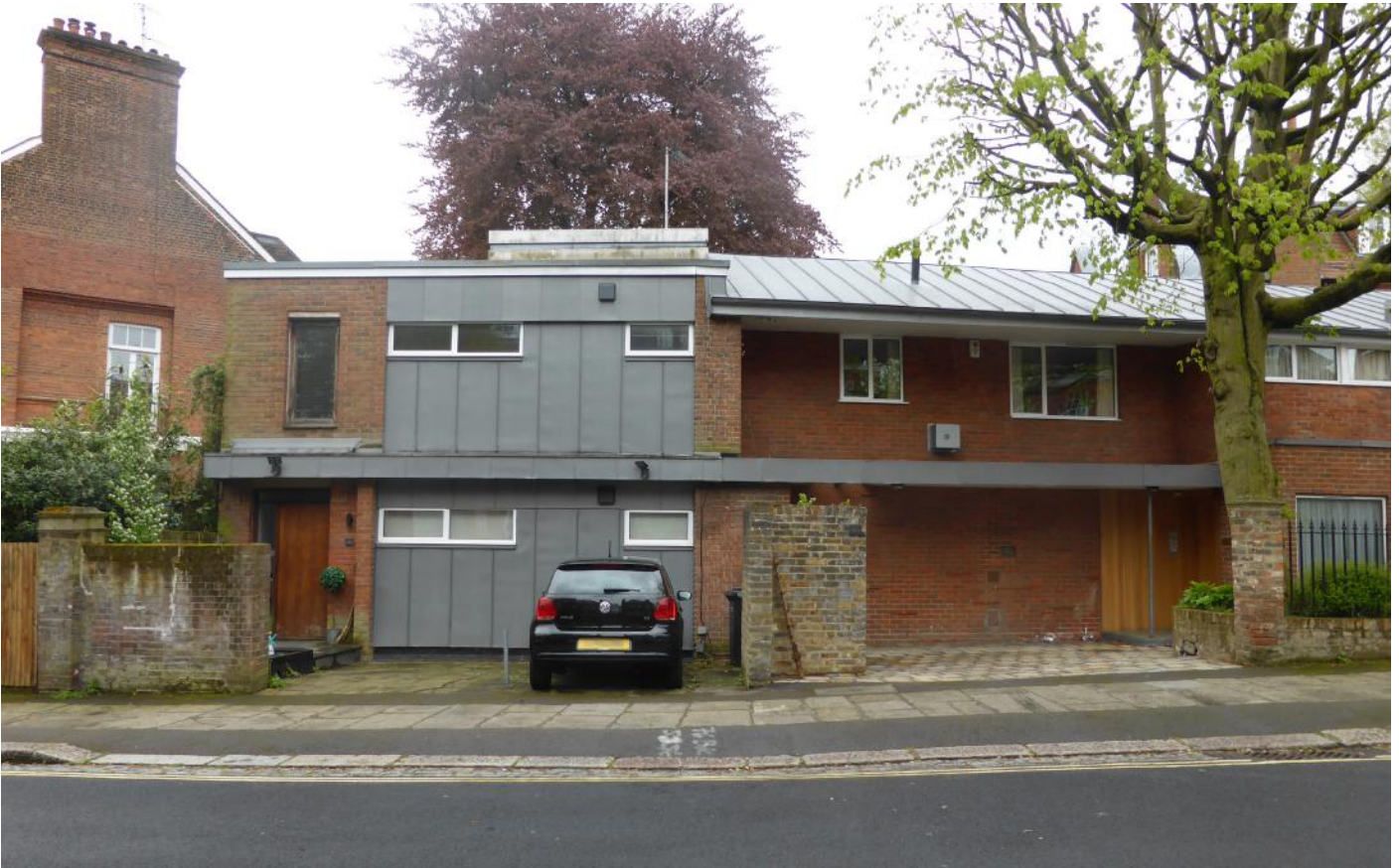
Figure 20: Photograph of the existing 4b exhibiting clumsy relationship with 4a at roof levels, small windows to north elevation
