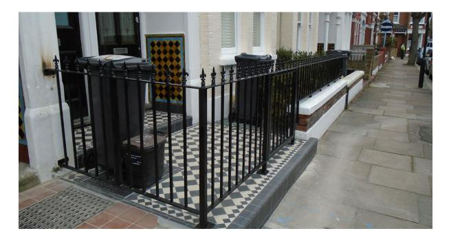
These are railings and accompanying gate that ARC manufactured and fitted in 2016 for a customer in Clapham, south-west London. They are mild steel railings with cast finials.
