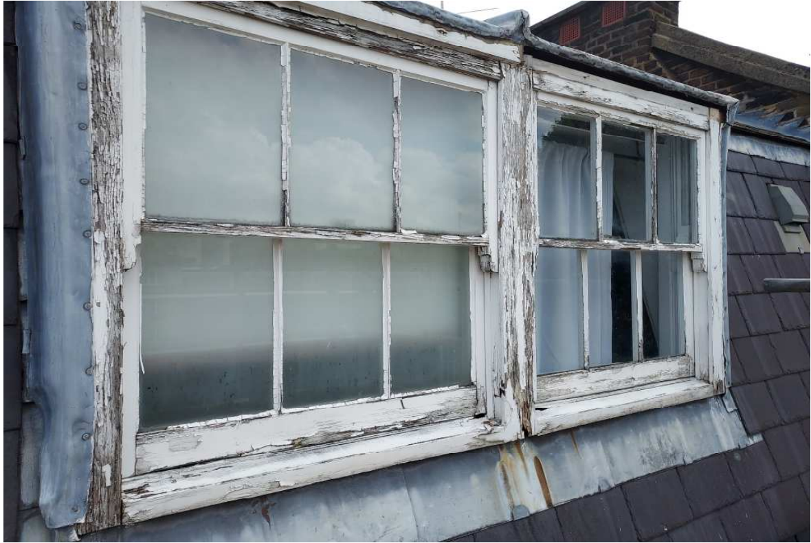
Figure 1: Timber sash window to be replaced.
