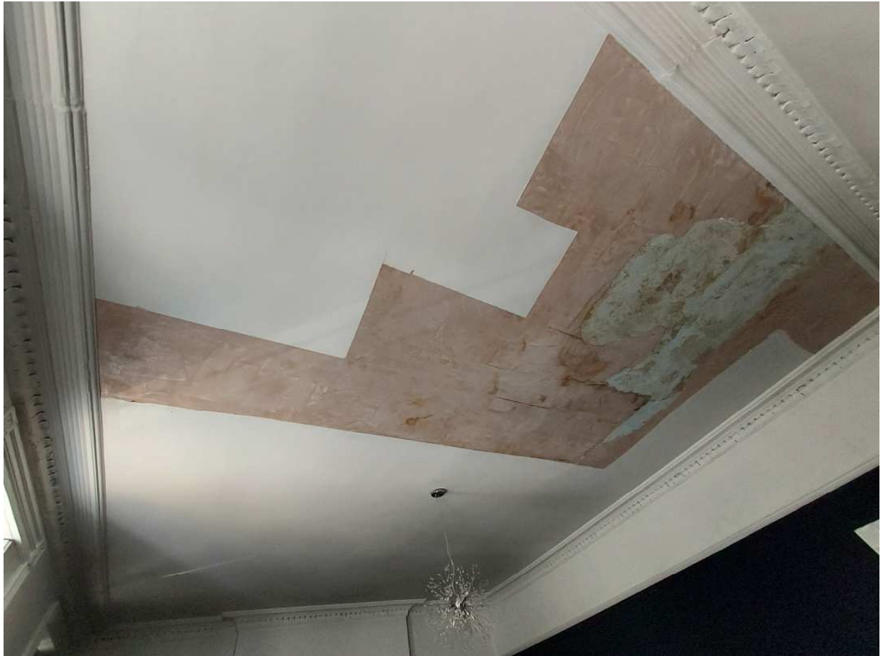
Figure 2: Location of ceiling to be replaced.
