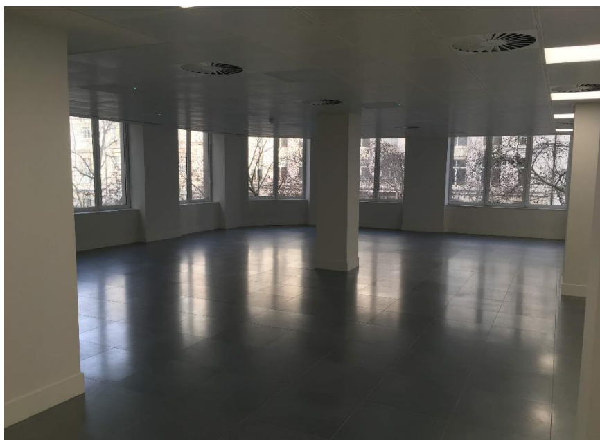
Figure 13 Typical interior of the upper floor office spaces (2019), there are no decorative features of interest, with columns encased in extensive layers of cladding. Note contrast in thickness between the columns seen to today to that of the historic photograph and shows within the plans.
