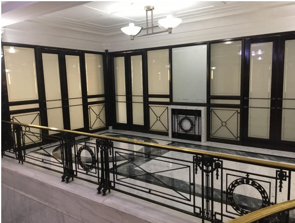
Figure 24 Interior of the principal entry hall at first floor level (2019). Note repositioned elements of the balustrade and modern glazed screening to the board room.
