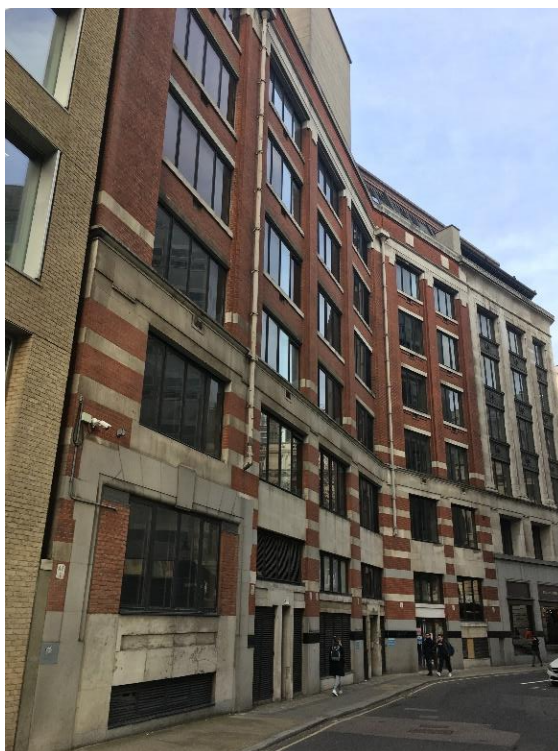
Figure 12 View of the Keeley Street elevation (2019). Note blocked secondary entrances.
