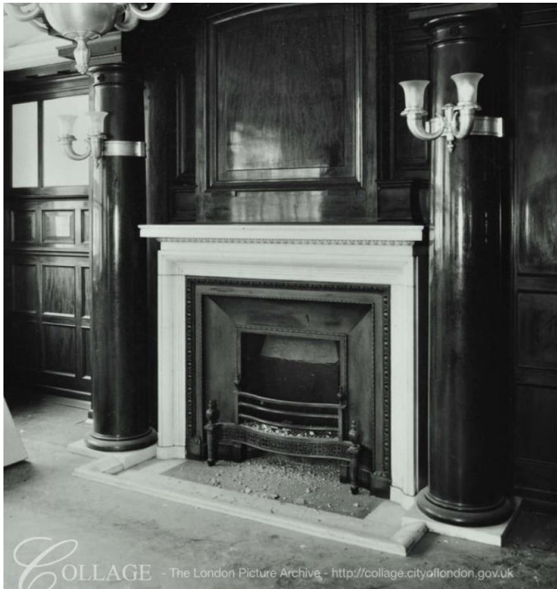
Figure 15 The fireplace within the first floor boardroom 1972 (Collage)
