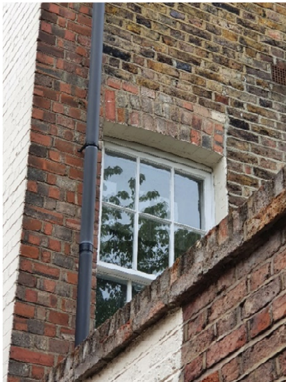
Poor unmatched brickwork to No10
