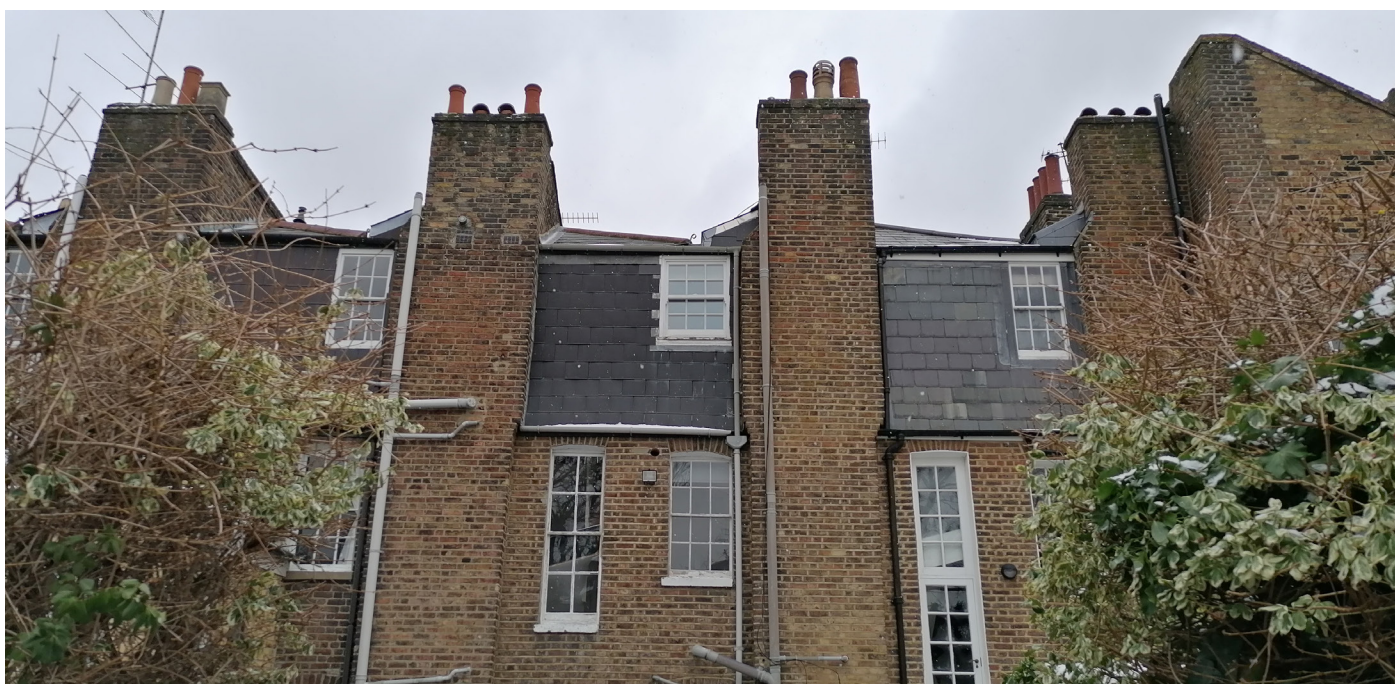
Photo 11. Rear elevation showing non-original 2nd floor sash window within slates. We aim to reinstate the original proportions of this window as still extant on the two adjacent houses.
